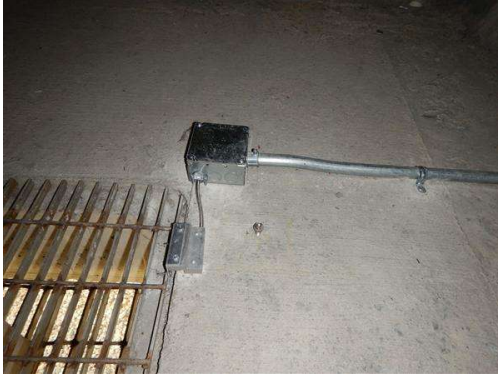
Photo 1 Security system was attached to the access hatch at Pier 1A
