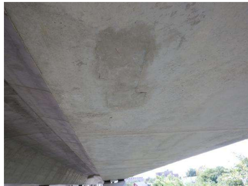
Photo 4 Concrete patches in the bottom flange of Spans 13A & 14A
