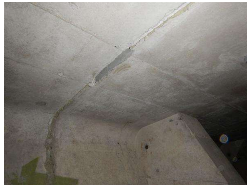
Photo 10 Concrete cut out of 20"x2.5"x5" in Segment 1A at Pier 17A at the shear key in the top slab
