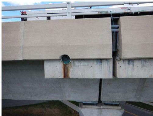
Photo 13 Drainage cap on the edge face of the end segment in Span 13A looking East
