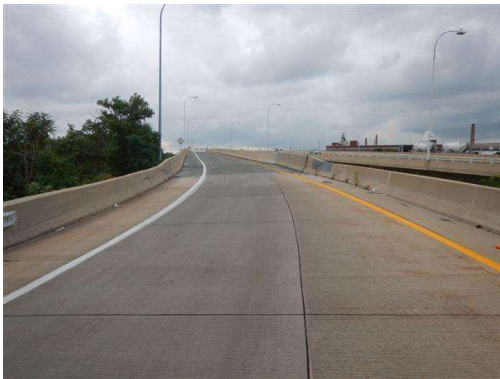
Photo 3 End View of Ramp D looking south.
