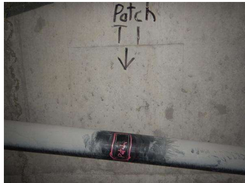
Photo 4 Patch added to the tendon in Span 7D due to previously documented gouge.
