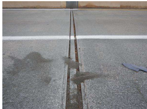
Photo 16 Typical condition of the expansion joints along the width of the roadway.
