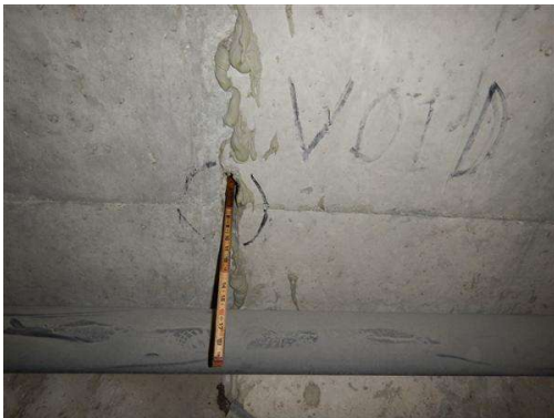
Photo 9 Typical interior void between segment joints.
