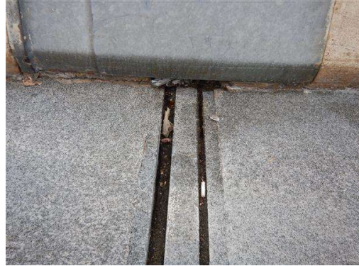
Photo 2 Foam filling void between barrier and approach slab at the west end of the expansion joint.
