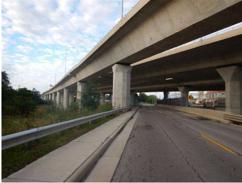
Photo 1 Ramp D Elevation View looking southwest.
