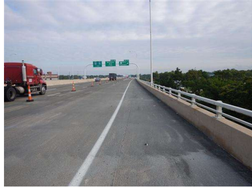
Photo 2 End View of Ramp D looking north.
