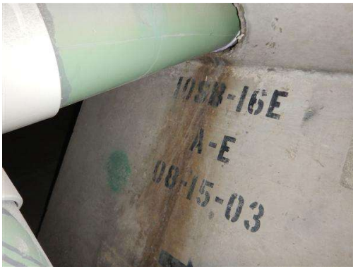
Photo 15 Interior drainage pipe at Pier 10SB
