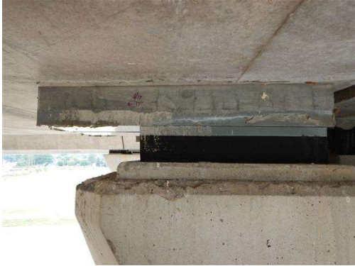
Photo 31 West bearing shifted 17" South at Pier 20SB
