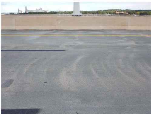
Photo 5 Lift hole patch with spall between Spans 24SB and 25SB
