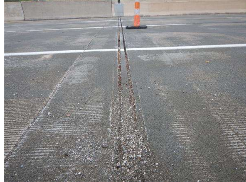
Photo 20 Expansion joint at Abutment 1NB looking West
