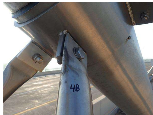
Photo 18 Welded repair to the West damper support at the lower sleeve cable clamp connections Cable Stay 4B
