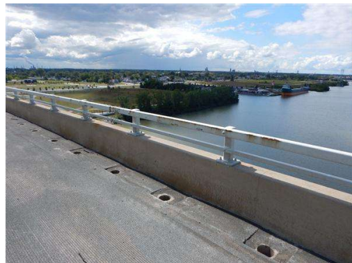
Photo 24 Typical condition of the steel railing along the length of the bridge
