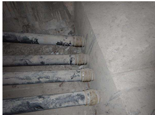
Photo 6 Soft PT tendon sleeves at Pier 26NB
