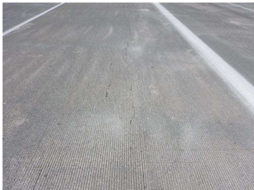
Photo 1 Transverse and map cracks along longitudinal joint in Span 46SB
