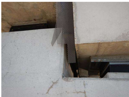
Photo 5 Hanging bird screen on the West face of Pier 30SB
