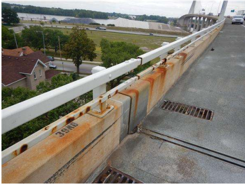
Photo 19 Typical condition of the steel railing along the length of the bridge looking South
