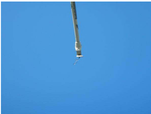
Photo 5 Missing light in Span 35NB
