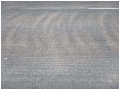
Photo 3 Transverse cracks at the segmental joint in Span 56NB
