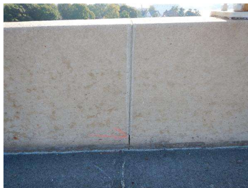
Photo 12 Bottom 2" saw cut in the East parapet unfilled looking East
