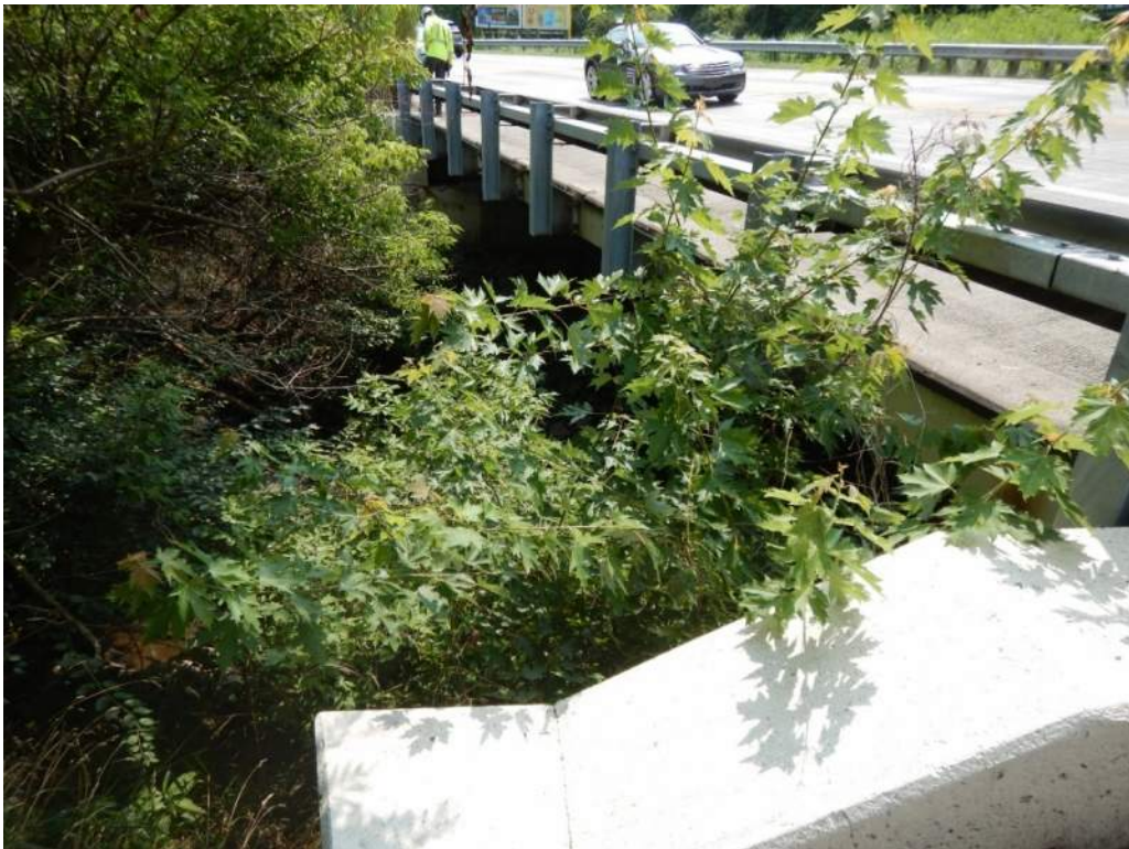
Upstream elevation of existing bridge
