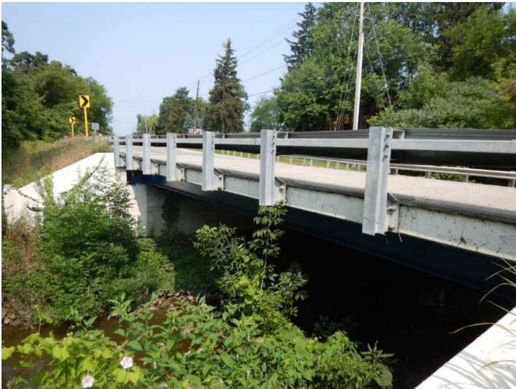
Downstream elevation of existing bridge
