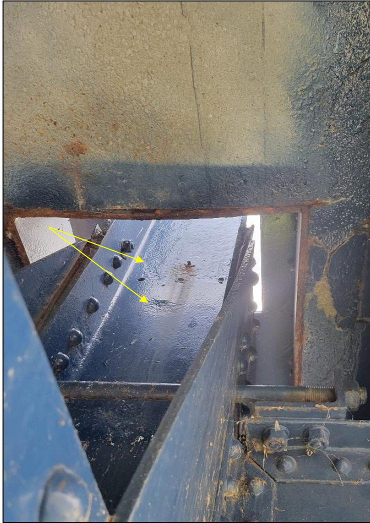
Picture 25: L8U8 of the north truss typical pitting in splash zone.
