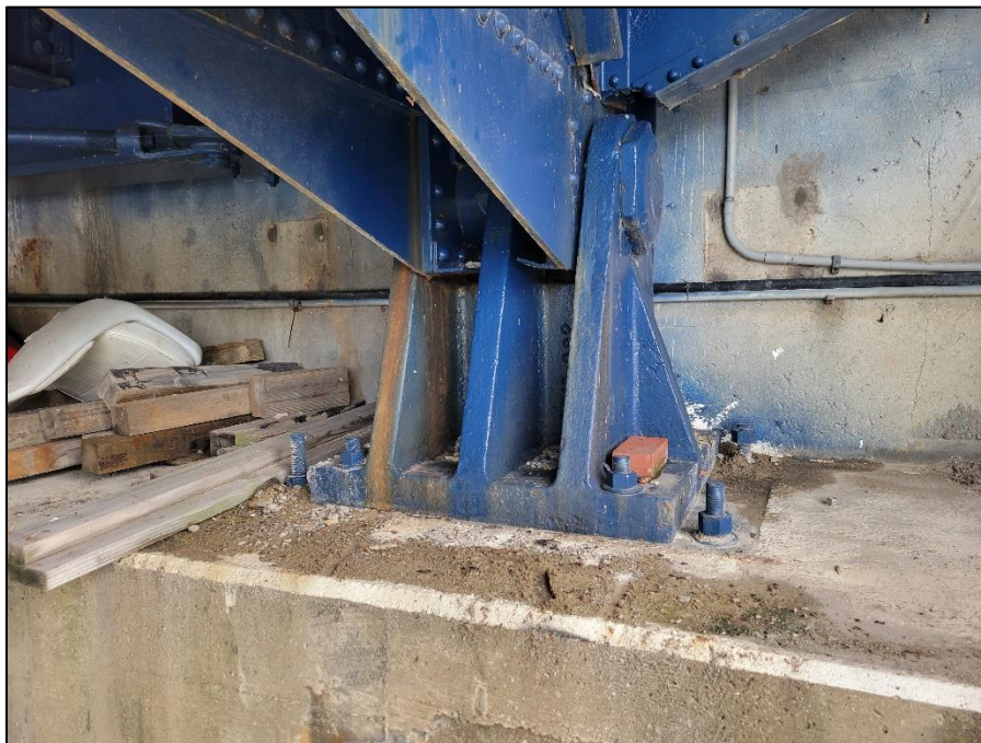
Picture 45: South bearing (bolster) on forward abutment.
