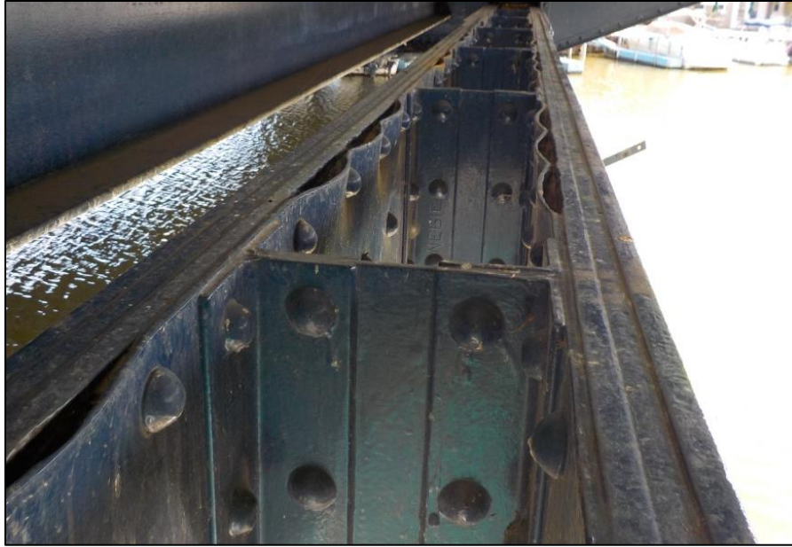
Picture 34: Pack rust in between plates of L3L4 of the south truss.
