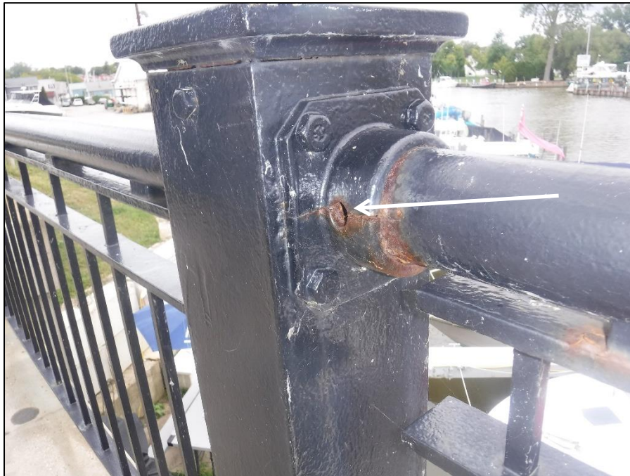
Picture 13: Missing bolt in connection plate.
