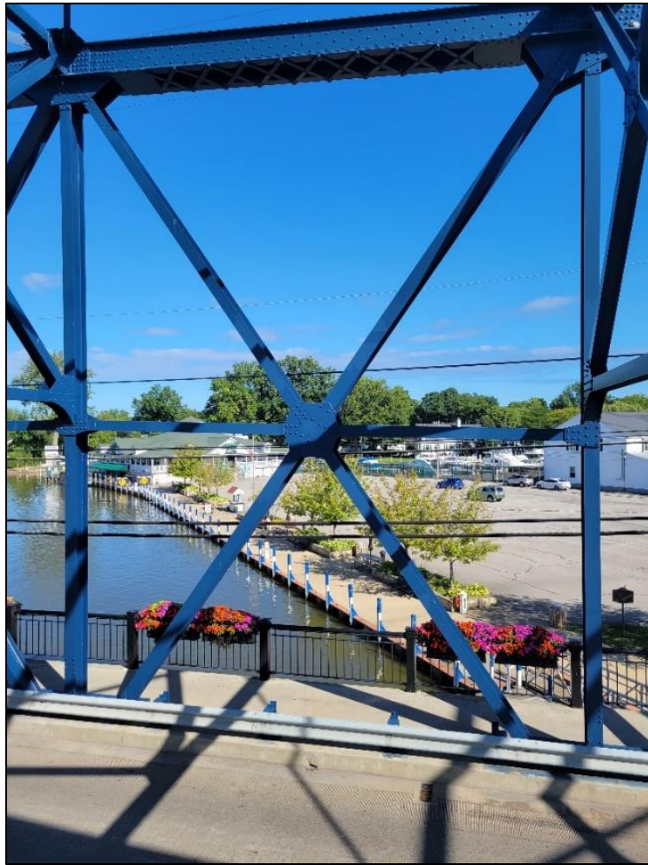
Picture 26: Typical X-diagonal (Panel 6 of north truss).
