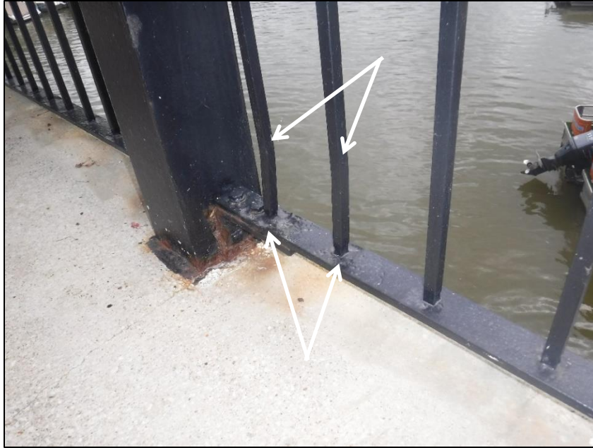
Picture 14: Bent vertical rails on pedestrian railing and section loss at bottom vertical rails.
