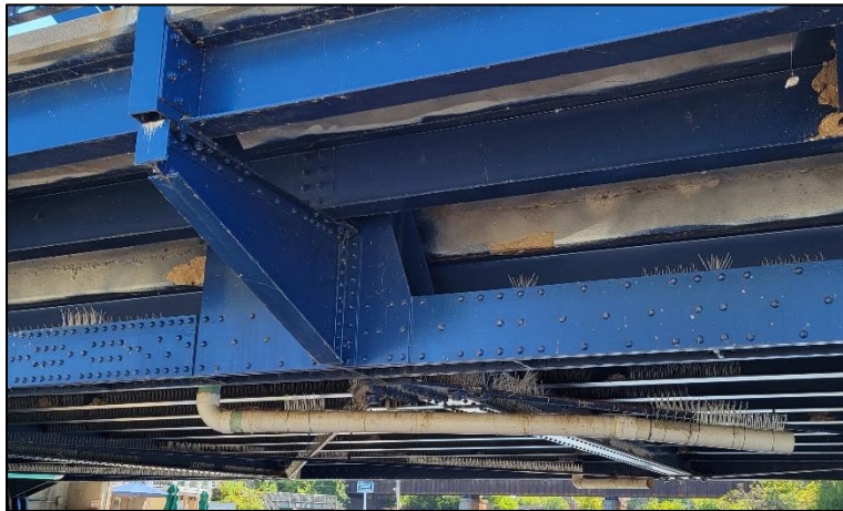
Picture 8: Typical sidewalk stringer condition.
