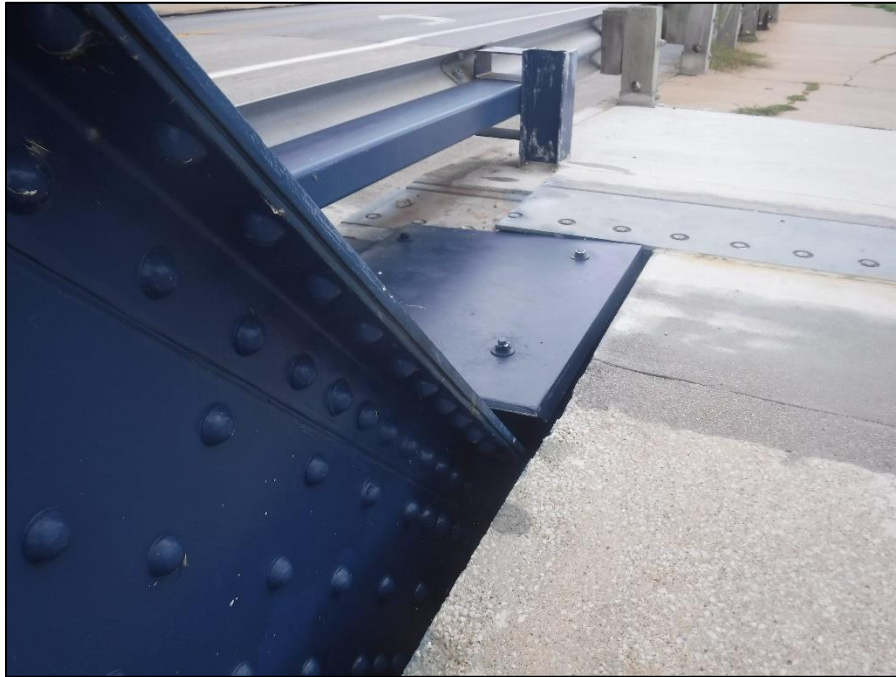
Picture 12: Minor misalignment of plates at L0 on north truss.
