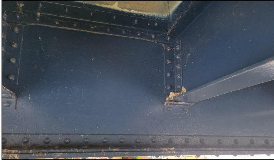
Picture 19: Typical bent stringer connection and support angle.
