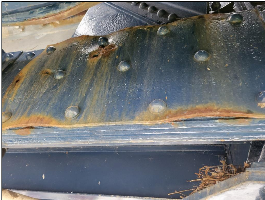
Picture 33: Holes in north inside plate of L5L6 at L6 of south truss.
