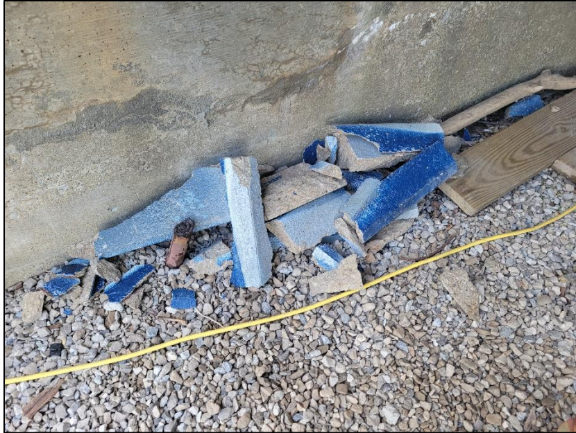
Picture 3: A portion of the spalls safely removed.
