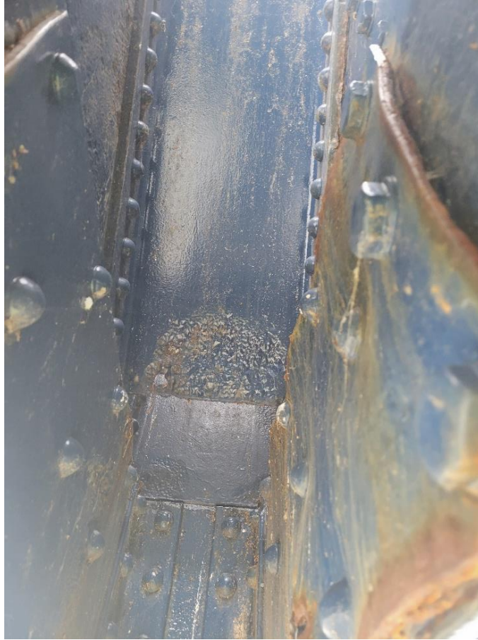
Picture 27: Reactivated pitting at the bottom of L7U8 of the south truss.
