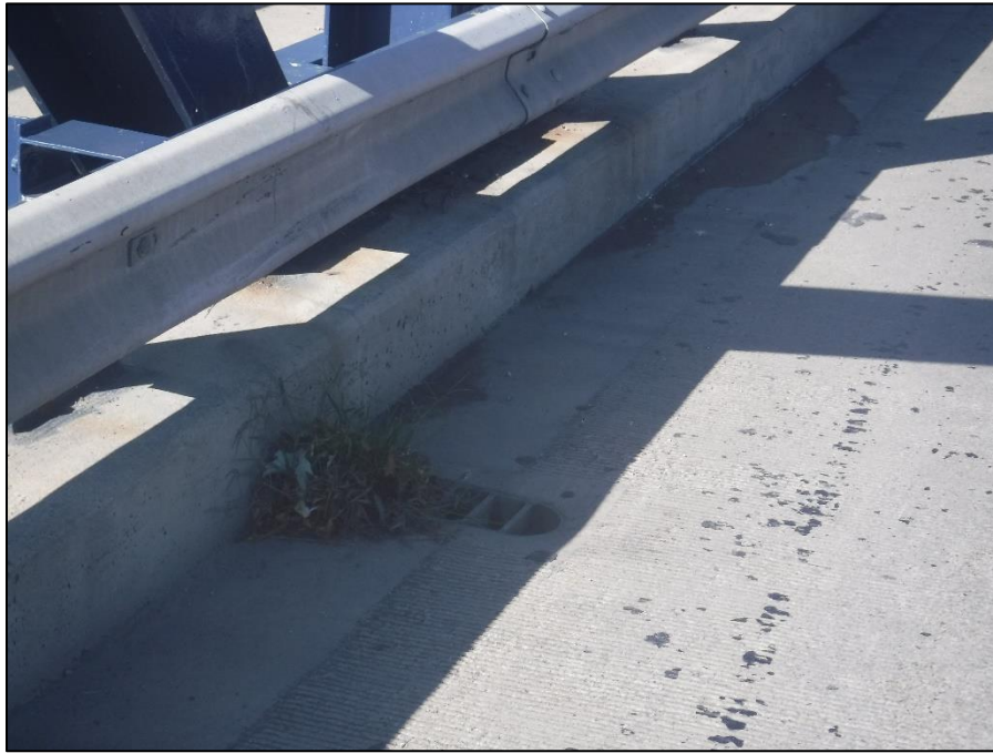
Picture 16: Evidence of ponding along south curb near L8 and partially blocked scupper.
