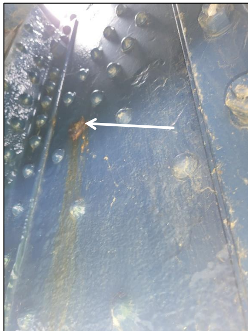
Picture 37: Looking at a rust hole through the inside gusset plate of L6 of the south truss.
