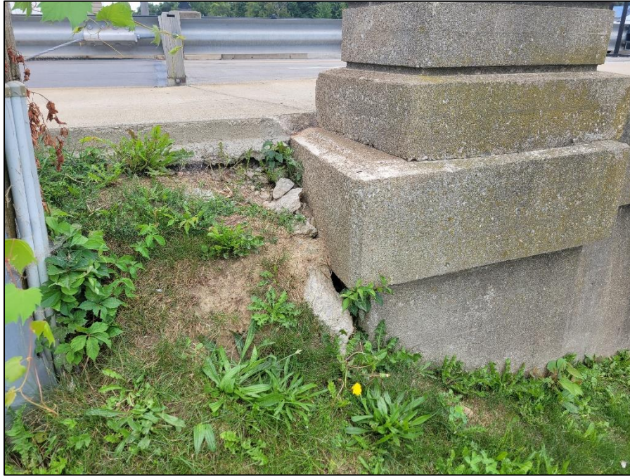
Picture 57: Erosion at northeast embankment is beneath sidewalk.
