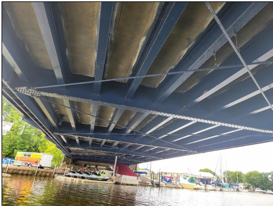
Picture 23: Typical floor system layout.
