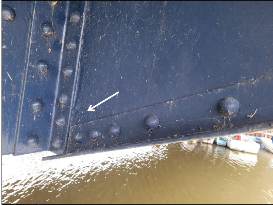
Picture 10: Looking east at pinholes in web of south cantilever bracket at L4.
