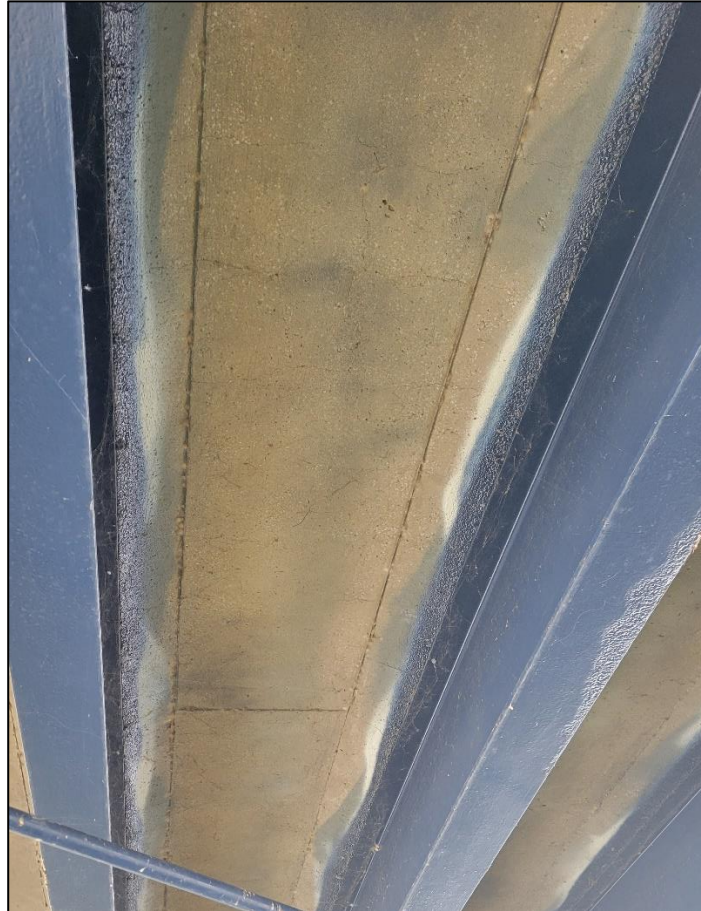
Picture 1: Typical hairline map cracking in deck.
