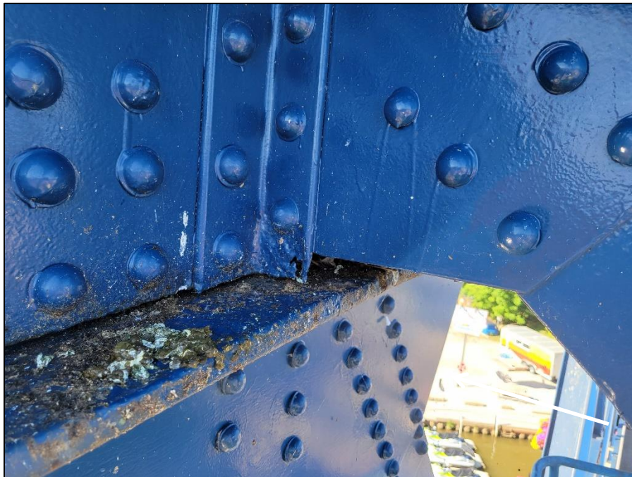
Picture 41: Looking west at sway brace connection to U6 of the south truss.
