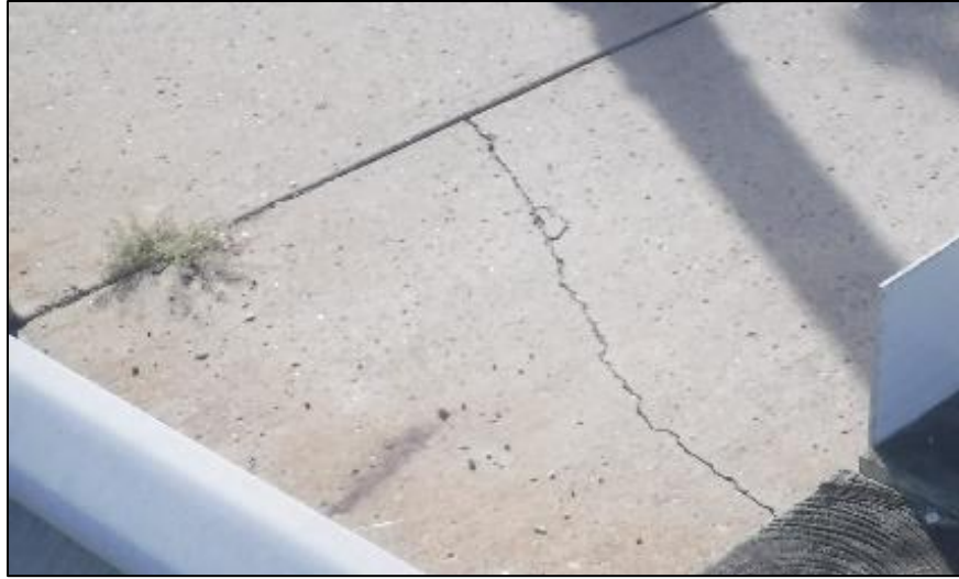
Picture 58: Approach sidewalk cracked at southwest corner.
