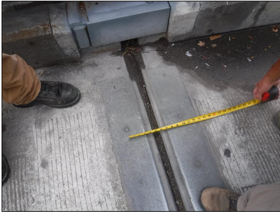
Picture 17: Expansion joint opening at rear abutment at north curb.
