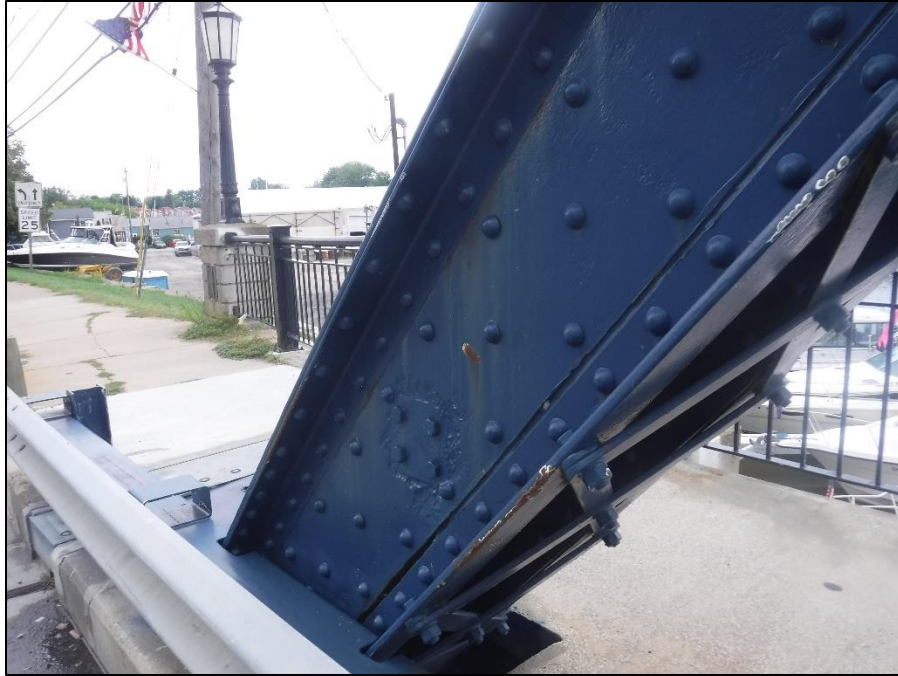
Picture 31: Looking at L0U1 of the north truss.
