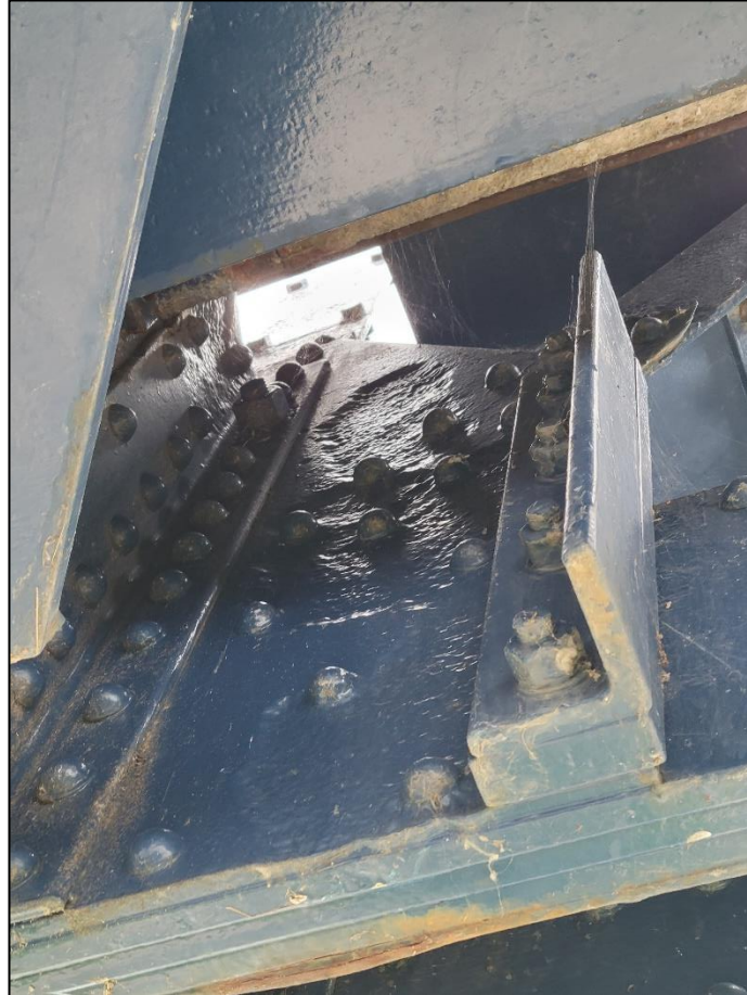
Picture 38: Looking at outside gusset plate of L4 of the south truss.
