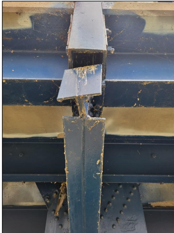
Picture 11: Bent south cantilever bracket.
