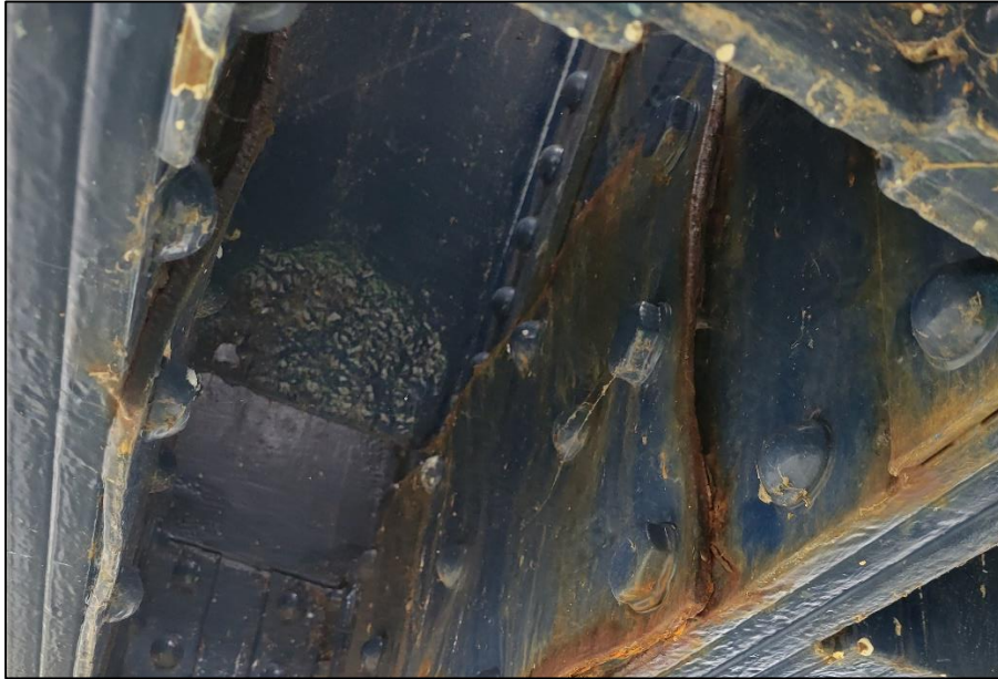
Picture 36: Pack Rust Bowing at L4 South Truss Inside Gusset Plate
