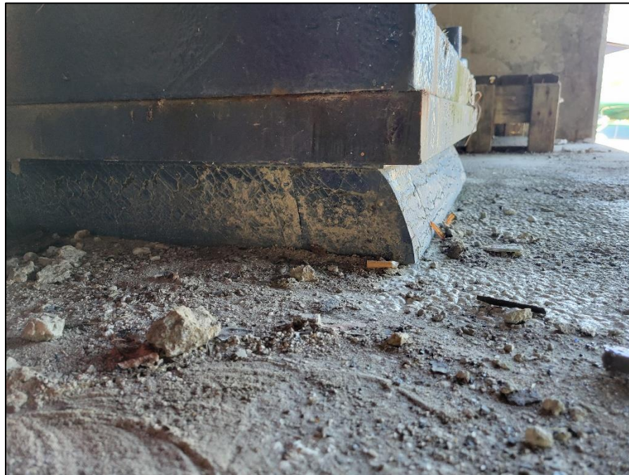
Picture 43: North elastomeric bearing on rear abutment.
