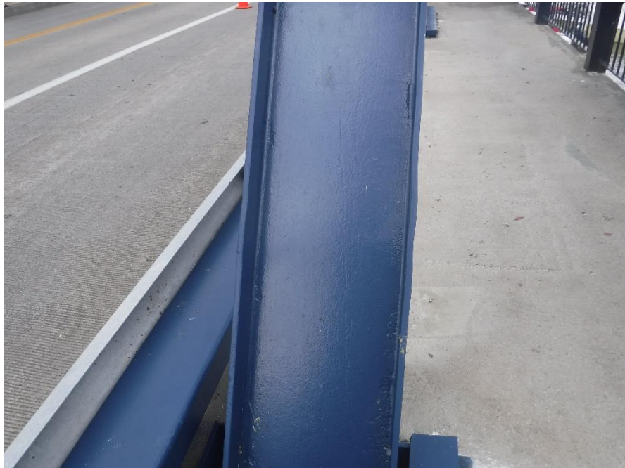
Picture 28: Minor waviness of north flange of U4L5 of the north truss.
