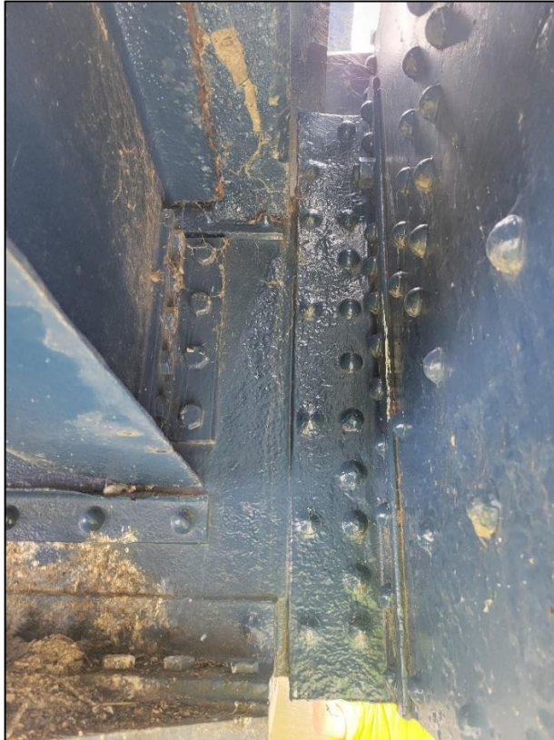
Picture 21: Floorbeam 5 truss connection plate; also, the stringer is not seated on the seat angle.
