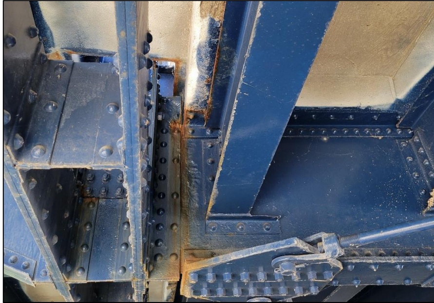
Picture 46: Floorbeam connection at L2 of the north truss.
