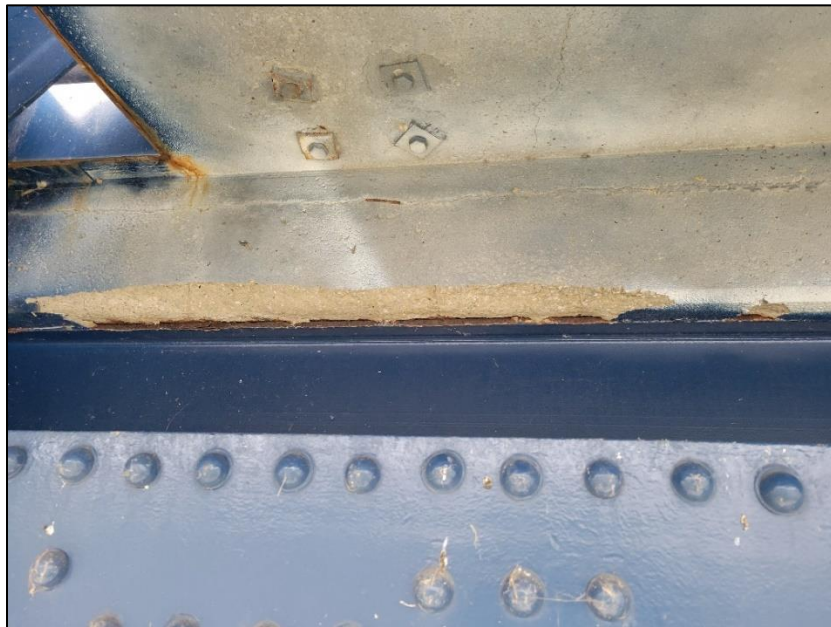
Picture 2: Spalls on south edge of deck in Panel 1.
