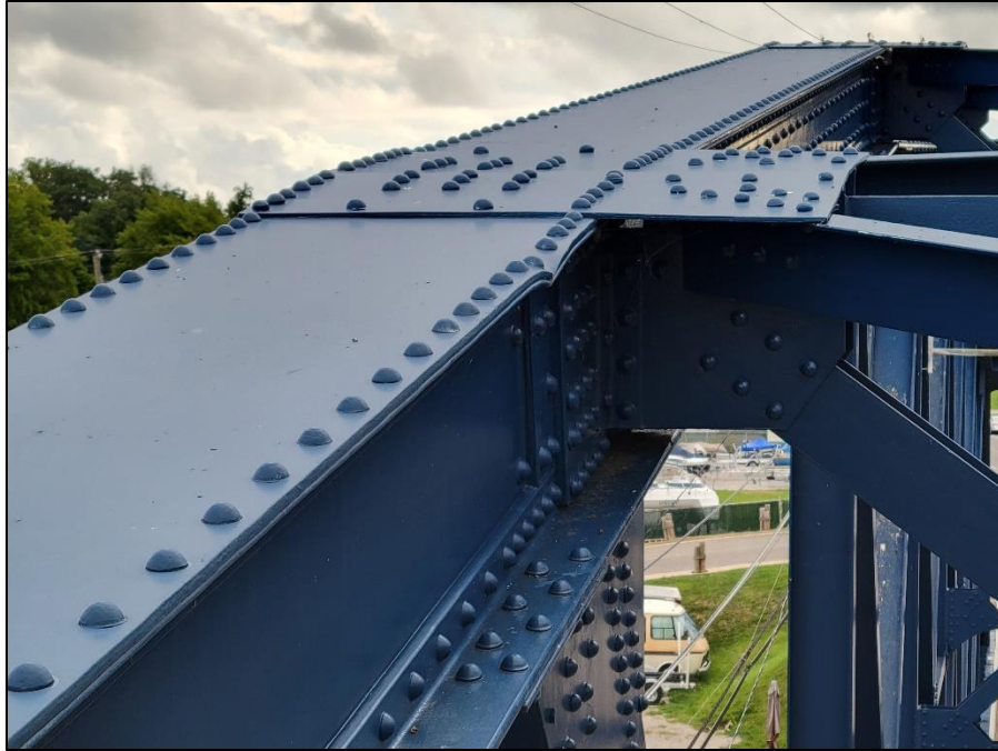
Picture 30: Dent in the top flange of U1U2 of the north truss.
