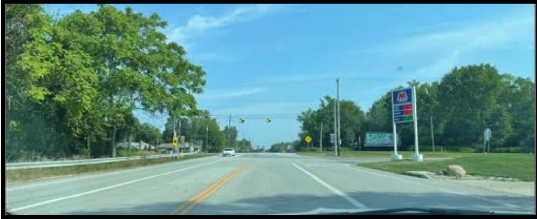
SR 57 Northbound approach
