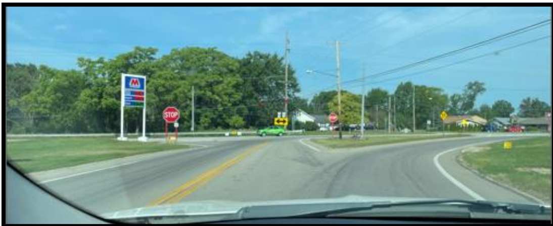
SR 82 Westbound approach (including Slip Lane to the right)
