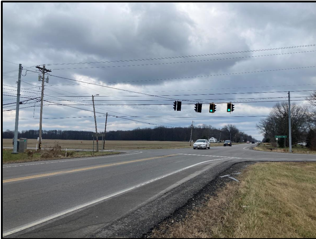
Image 1 – SR 82 & Durkee Road Signal from the southwest corner (January 2022)
