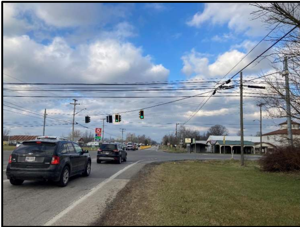
Image 1 – SR 82 & SR 83 Signal from the southeast corner (January 2022)
