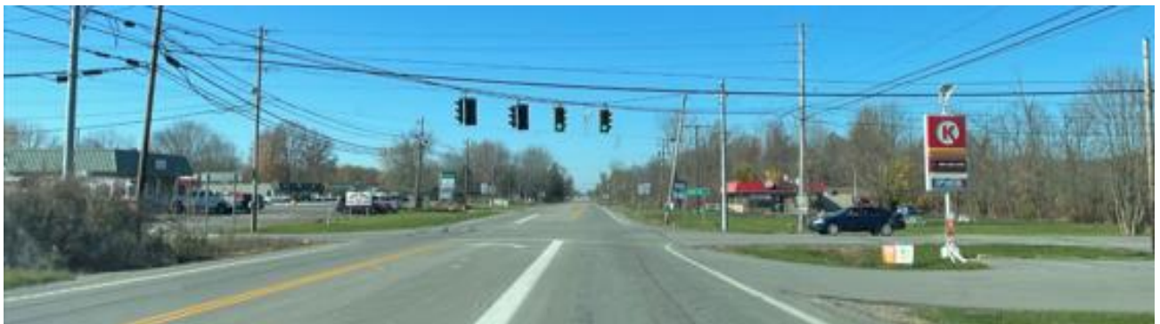
8. SR 82 WB 50 ft before stop line
