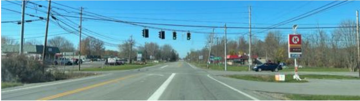
Figure 4. SR 82 westbound at the intersection
