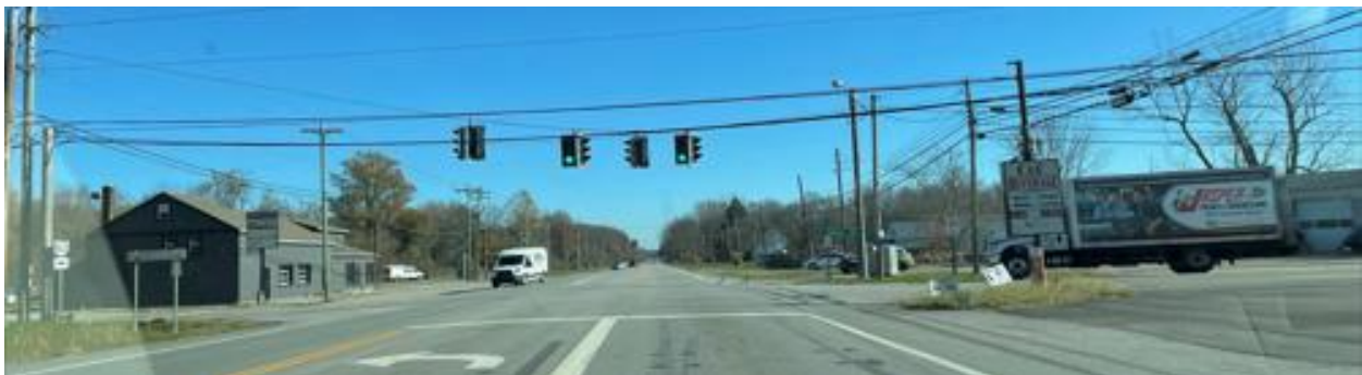
Figure 3. SR 82 eastbound at the intersection
