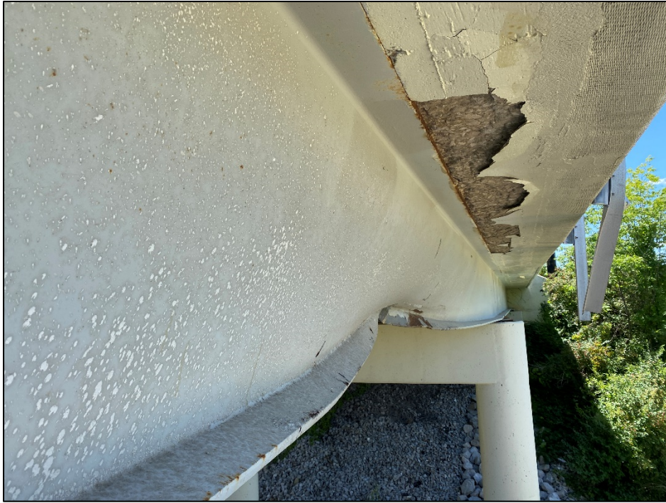
Photo # 3: Beam 1 alignment with respect to pier 1.
