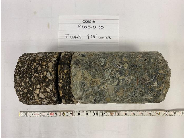
Project Name: SUM 76-77 Phase 3 Retaining Wall on SR8 Project Number: 1822-1016-00 Boring: P-005-0-20 Asphalt: 5" Concrete: 9.25" Date Cored: 06/26/2020 Date Drilled: 06/26/2020
