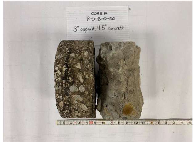
Project Name: SUM 76-77 Phase 3 Retaining Wall on SR8 Project Number: 1822-1016-00 Boring: P-018-0-20 Asphalt: 3" Concrete: 4.5" Date Cored: 06/24/2020 Date Drilled: 06/24/2020
