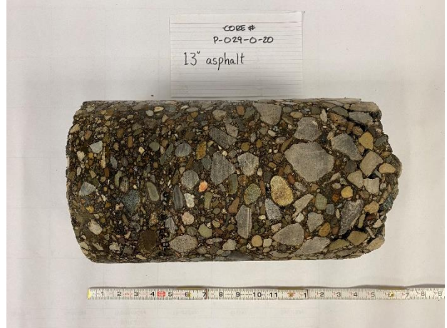
Project Name: SUM 76-77 Phase 3 Retaining Wall on SR8 Project Number: 1822-1016-00 Boring: P-029-0-20 Asphalt: 13" Concrete: Date Cored: 06/22/2020 Date Drilled: 06/22/2020
