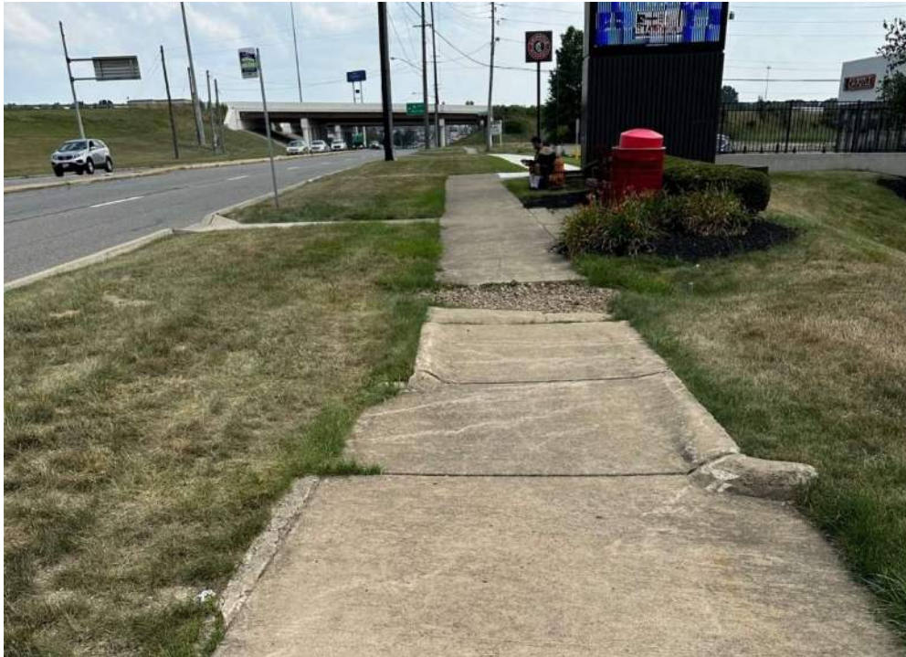
Figure 11. Jagged and missing sidewalk on the west side of Belmont Avenue between Liberty Street and the I-80 westbound ramps
