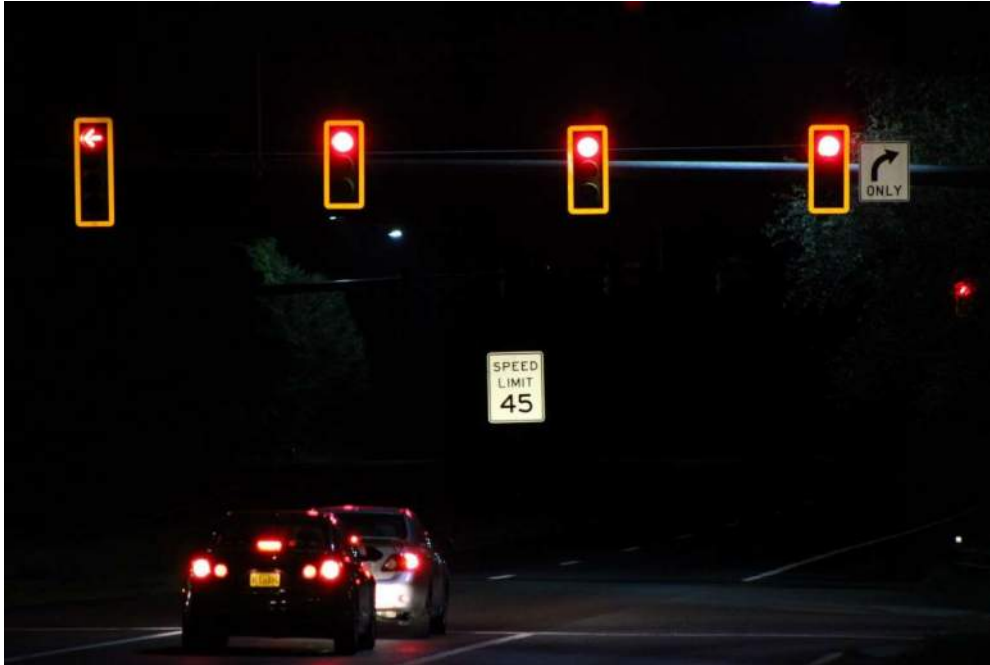
Figure 52. Reflective signal backplates increase signal visibility during dark hours
