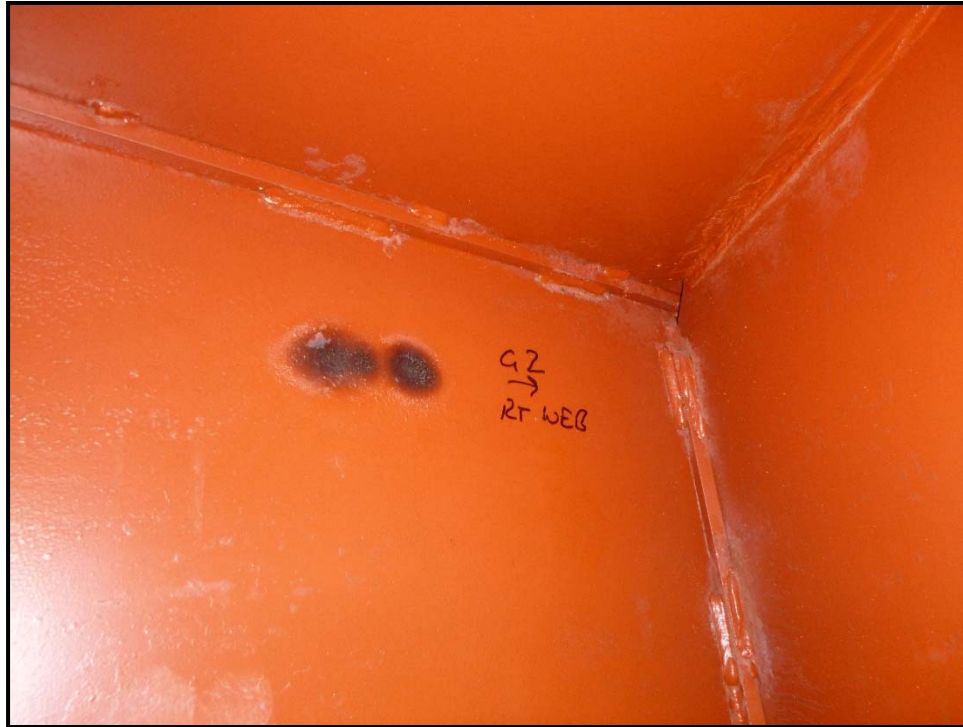
Photo 23 – STA-77-0912 – Fatigue Prone Detail #3, no distress observed
