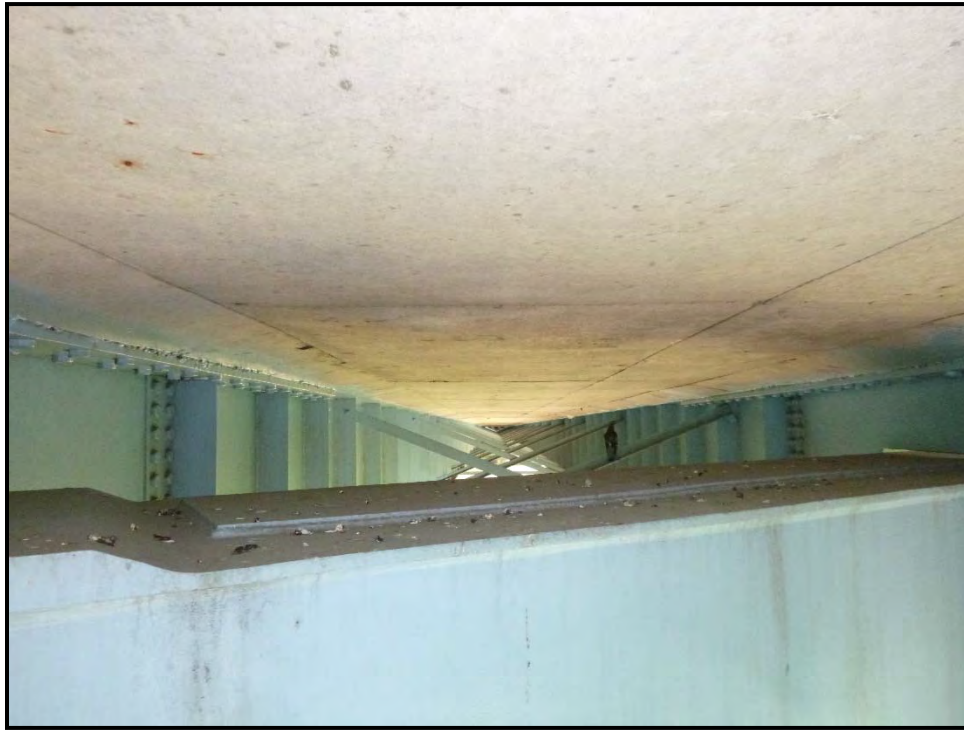
Photo 26 – STA-77-0912 – Fatigue Prone Detail #7, no distress observed.
