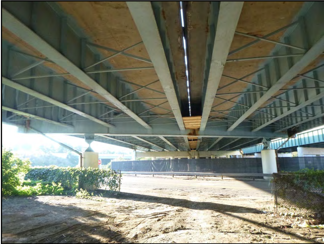
Photo 1 – STA-77-0912 – Integral steel box girder (Pier #3), Looking South
