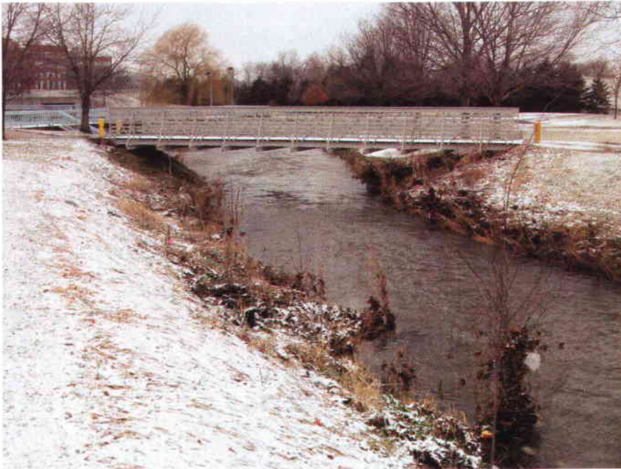
Photo 2 – Downstream Side of Pedestrian Bridge (looking east)
