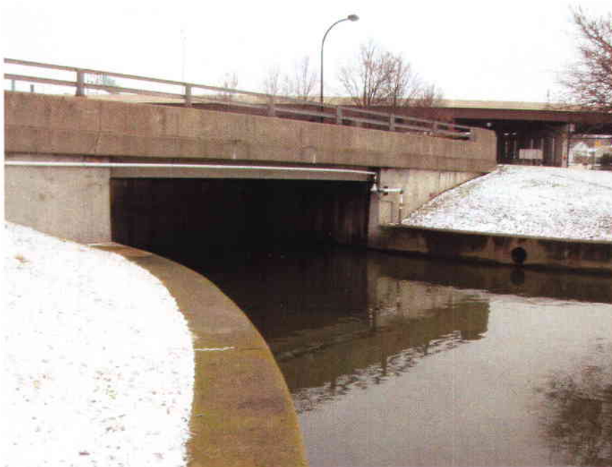
Photo 4 – Downstream Side of Kelly Avenue Bridge (looking southeast)
