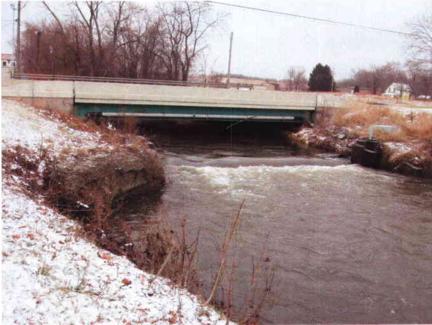
Photo 5 – Downstream Side of Seiberling Street Bridge (looking east)
