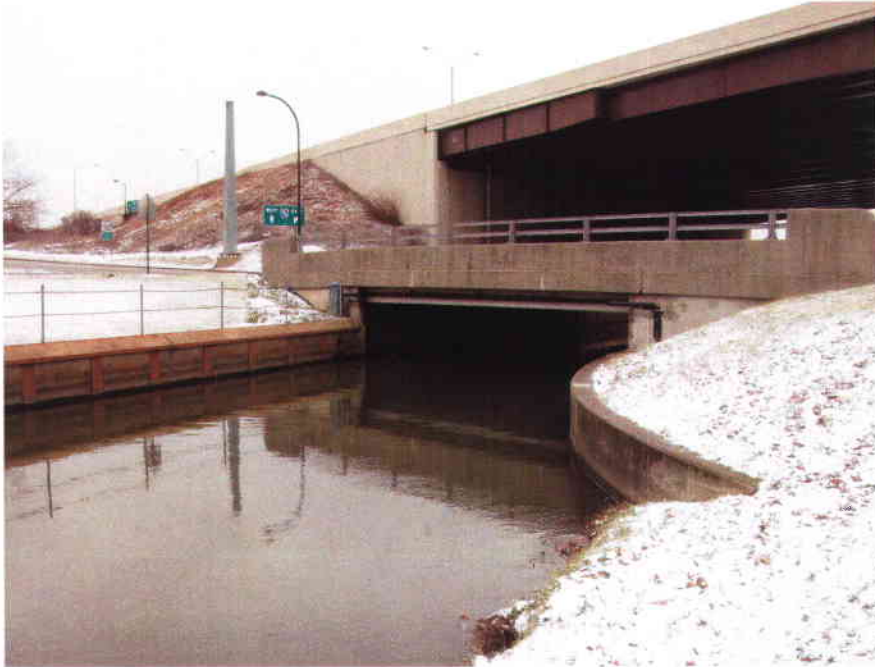
Photo 3 – Downstream Side of 3 rd Avenue Bridge (looking southeast)
