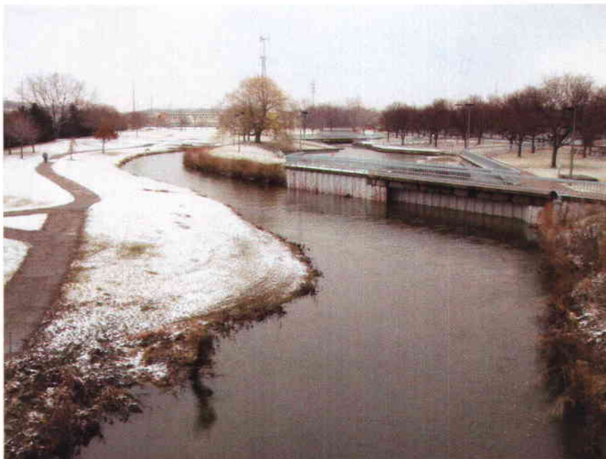
Photo 6 – Relocated River in Middlebury Run Park (at Martha Ave. looking east)
