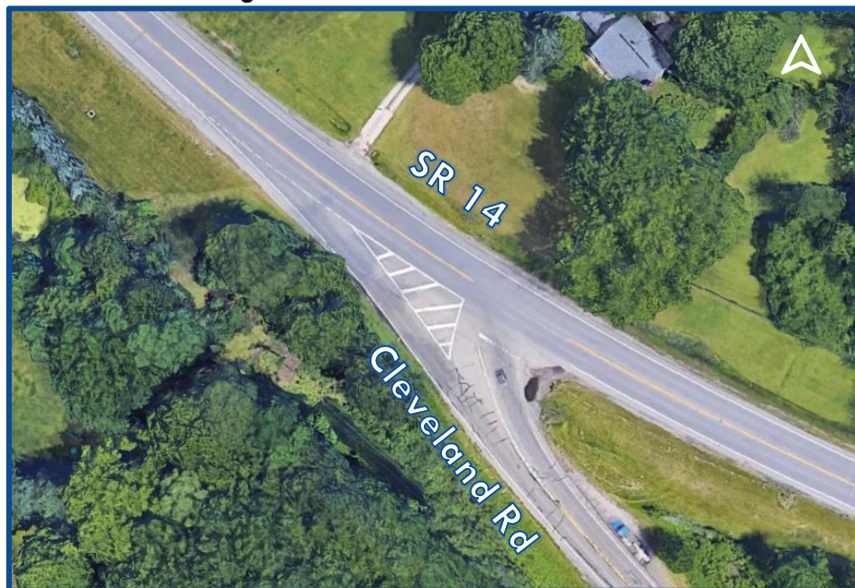
Figure 4: SR 14 and Cleveland Road
