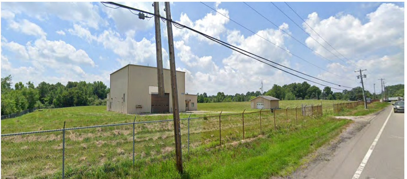
Photograph 2: Site RM-004. Viewing groundwater recover building, looking southwest.
