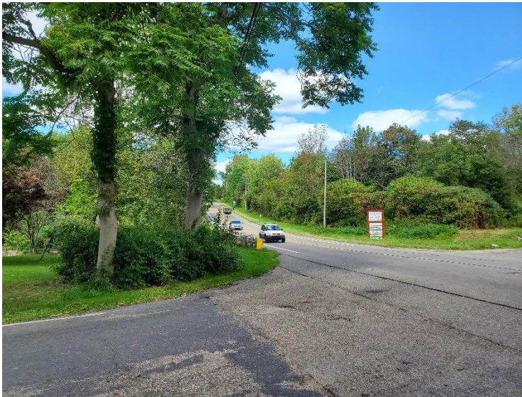
Photo 1: Randolph Road Eastbound Approach Looking North (Photo taken 9/23/2022)
