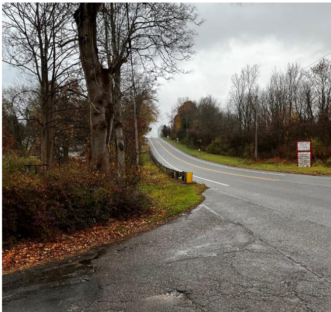
Photo 2: Randolph Road Eastbound Approach Looking North (Photo taken 11/5/2021)
