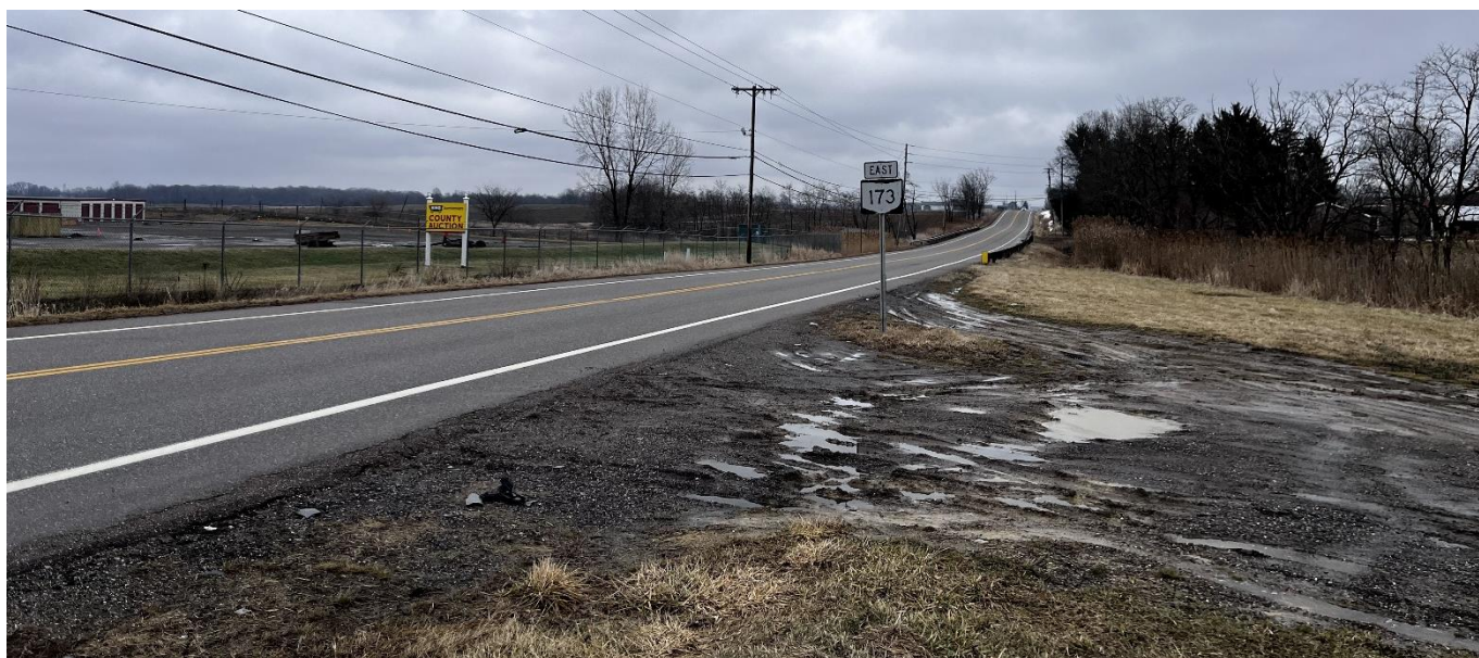
Figure 2 - Southeast Quadrant Gravel Area
