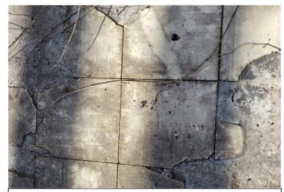
Photo 2 – View of asbestos-containing tan floor tile in concrete structure.
