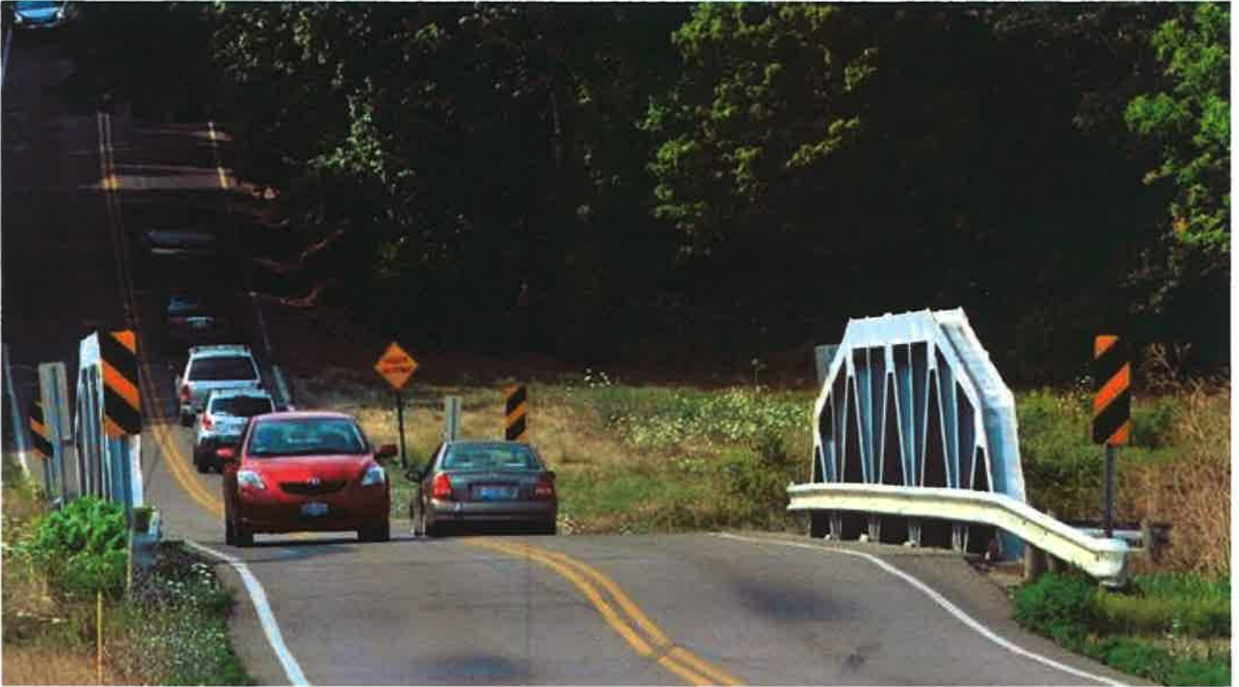
Vehicles drive on a bridge Wednesday on Ety Road in Lancaster. City and county officials are looking at developing a plan to replace the two bridges on the road. / Matthew Berry/ Eagle-Gazette
