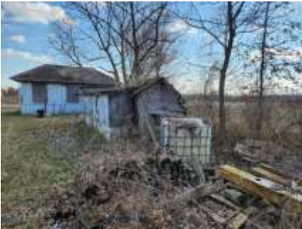
View of Building No. 3 and Parcel 36 looking east
