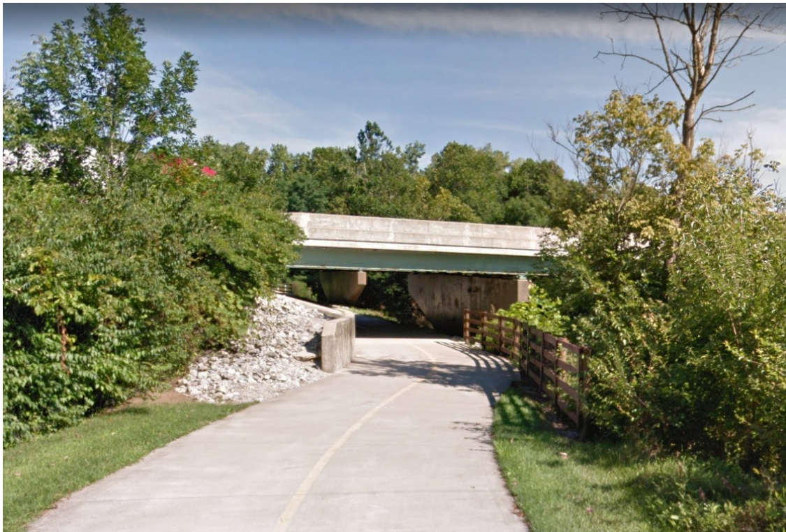
Temporary impacts to the Blacklick Trail running under IR 70 are likely during construction
