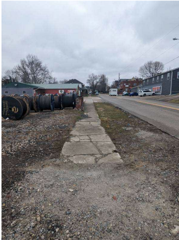
Photo 2: Existing infrastructure along the corridor that is in poor condition. Source: OMEGA
