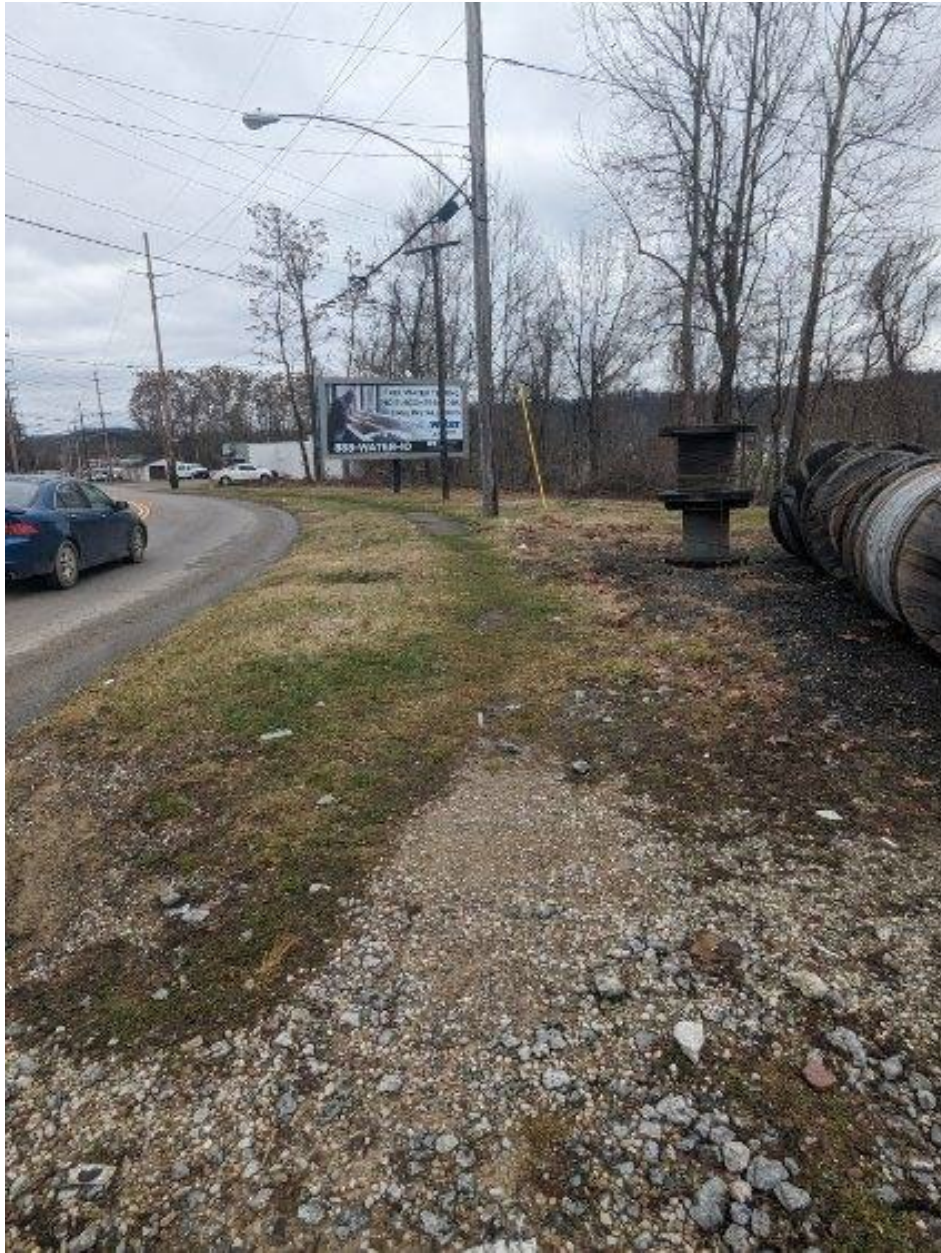
Photo 1: Lack of pedestrian infrastructure along S. 11 th Street (Goat Path)
