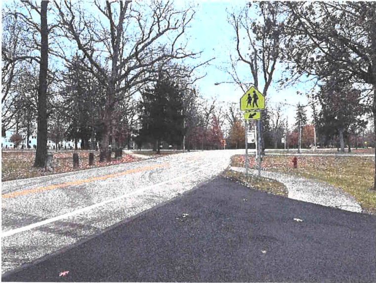
Chase Avenue Crossing
