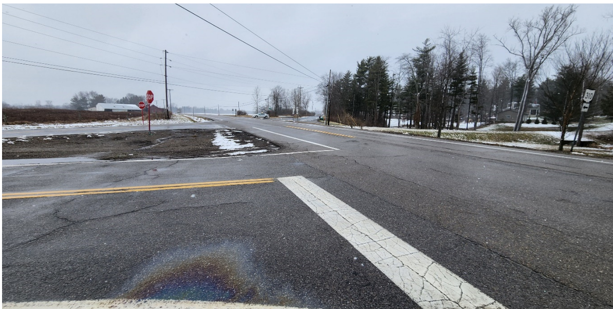
Figure 2: SR 37/SR 310/Windy Hollow Road intersection (looking NNW)
