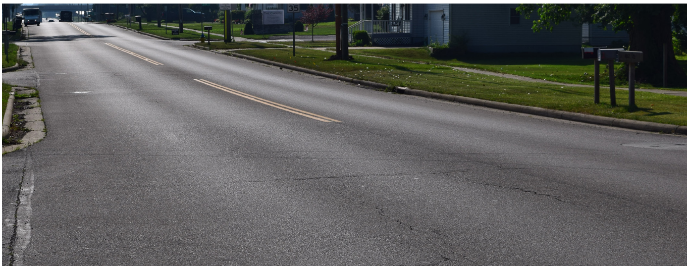
Figure 6: At 36', Main Street is very wide for a two lane roadway
