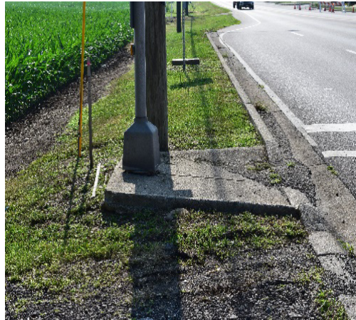
Figure 1: The crossing cutout on the north side of US-40 across from Arrowhead Drive is unconnected to any sidewalk on from either side
