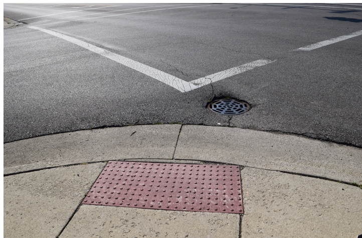
Figure 3: Single cut curb crossing with truncated dome facing into middle of High and Main Streets intersection
