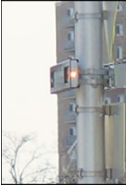
Figure 2. View of pilot light to pedestrian at shared-use path crossing with median refuge. Enlargement of pilot light at right.
