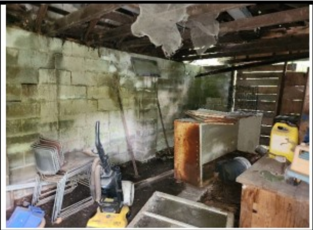
Interior view of outbuilding
