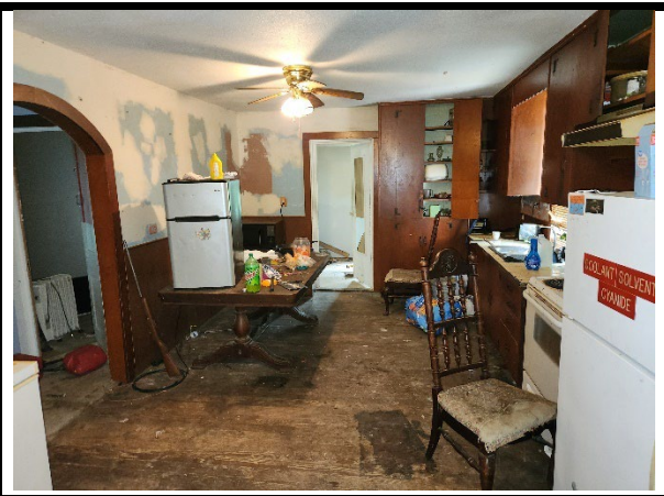
View of kitchen
