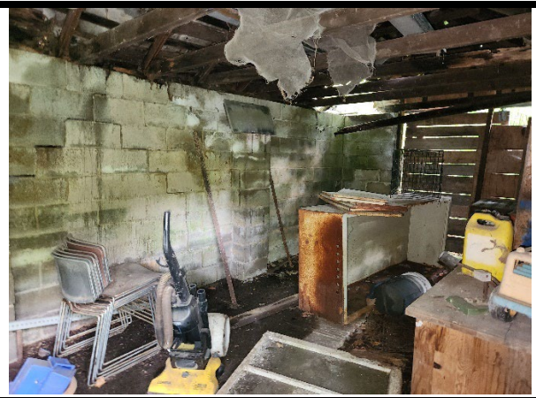
Interior view of outbuilding
