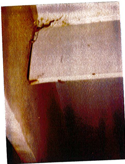
Bm #1 Stiffener on Inside
