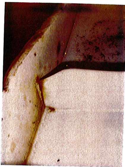
Bm # 1 Stiffener Rear of Impact
