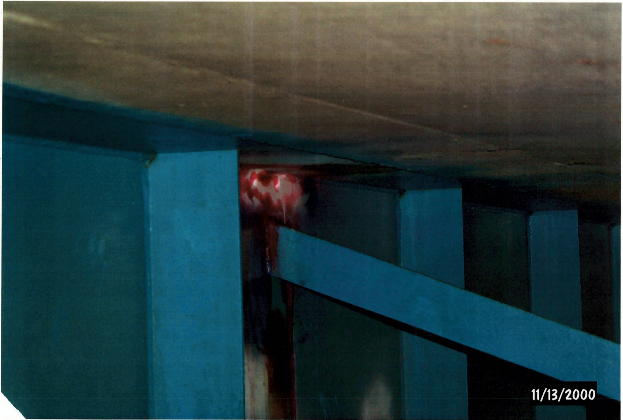
CRACK LOCATION #2 WITH \frac{3}{4} " HOLES DRILLED
