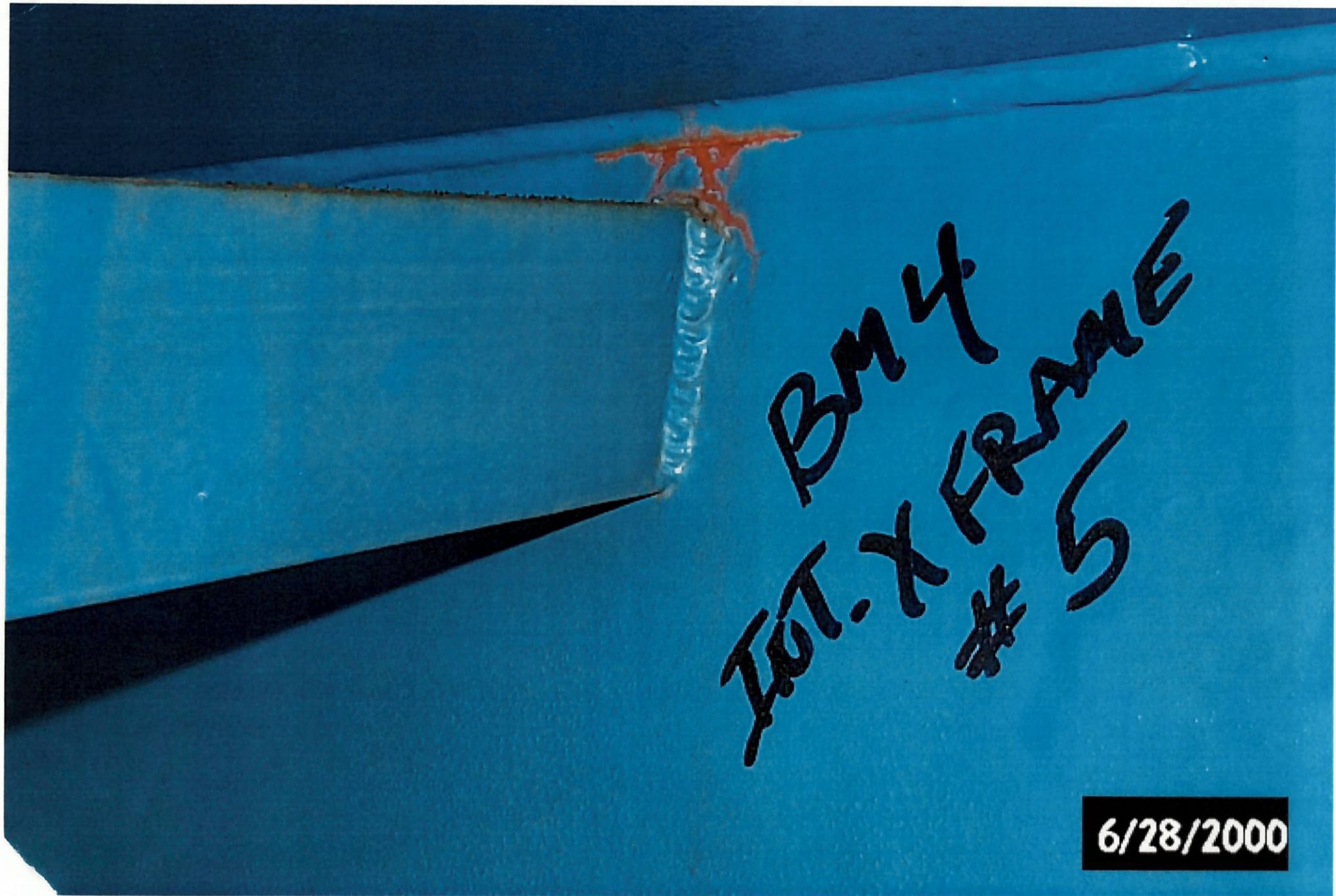
CRACK LOCATION #2
