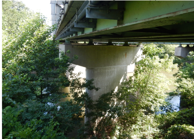
Pier View of 1.86L (Looking Northeast), 2017
