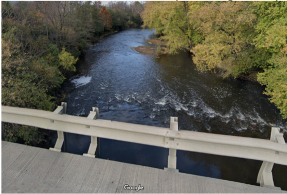
FRA-CR 122-1.86L (Looking West)
