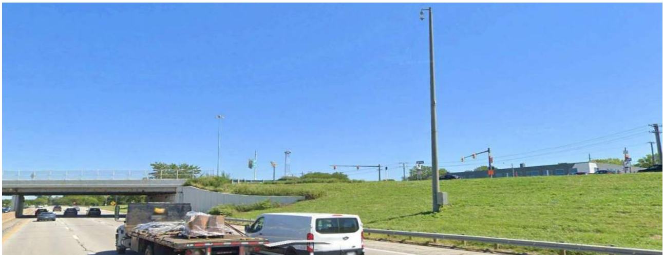
Figure 68: QWS-OVRHD-D12-I-90_WB AT DOWNTOWN Street view of DMS sign and structure to be replaced with new detection camera
