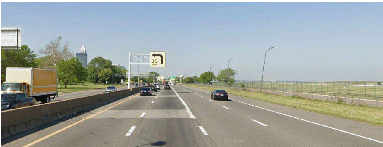
Figure 64: QWS-OVRHD-D12-I-90_WB AT DOWNTOWN Street view of replacement structure, new DMS, and new detection camera on existing CCTV pole
