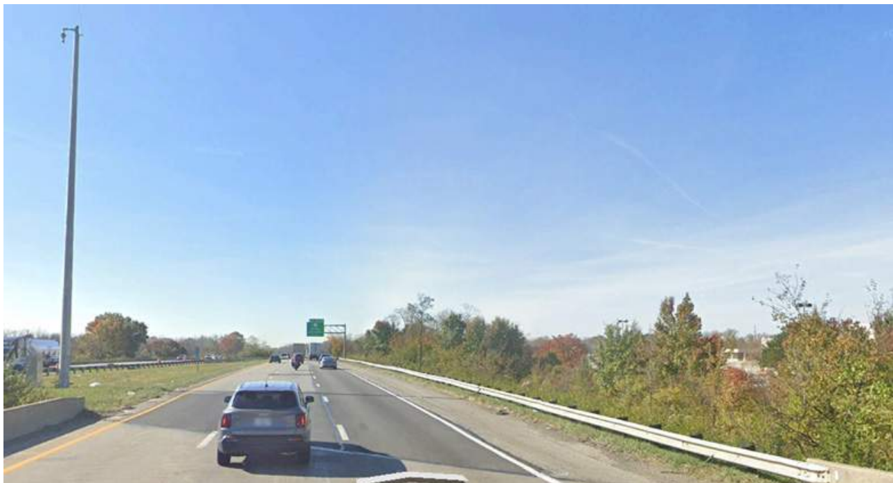
Figure 25: QWS-GRND-D6-I-270_SB AT SR 317 QWS Panel street view
