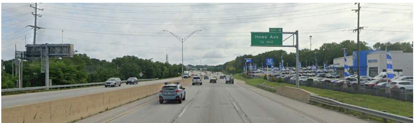
Figure 10: LITE-D4-OH-8_NB AT HOWE AVE Street view of proposed detection camera on existing SB DMS structure
