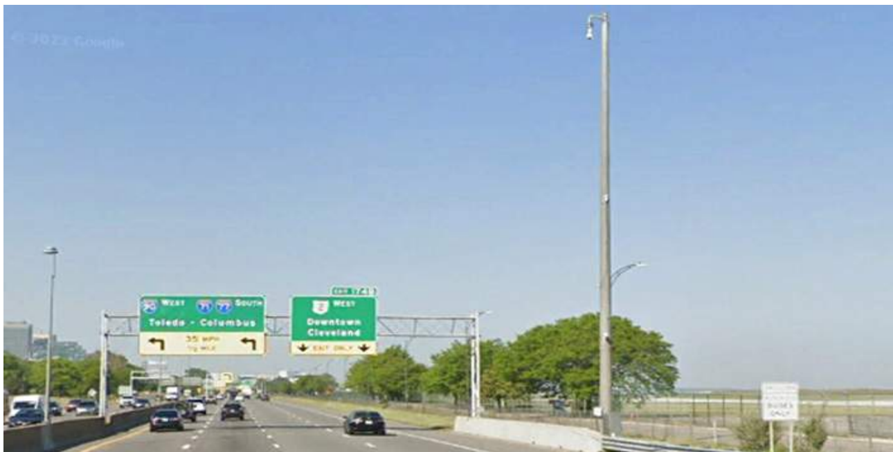
Figure 62: QWS-OVRHD-D12-I-90_WB AT DOWNTOWN Street view of replacement sign, new DMS, and new detection camera on existing CCTV pole
