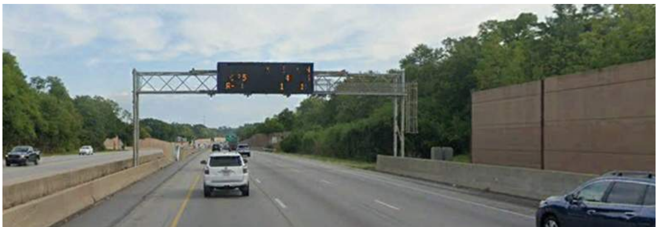
Figure 42: QWS-OVRHD-D8-I-71_SR 126 street view of proposed detection camera (with DMS to be replaced)
