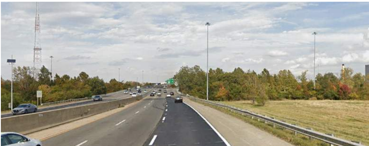
Figure 29: QWS-GRND-D6-I-670_EB AT SCIOTO RIVER BRIDGE street view of QWS panel at Scioto River Bridge at SLM 2.12 EB
