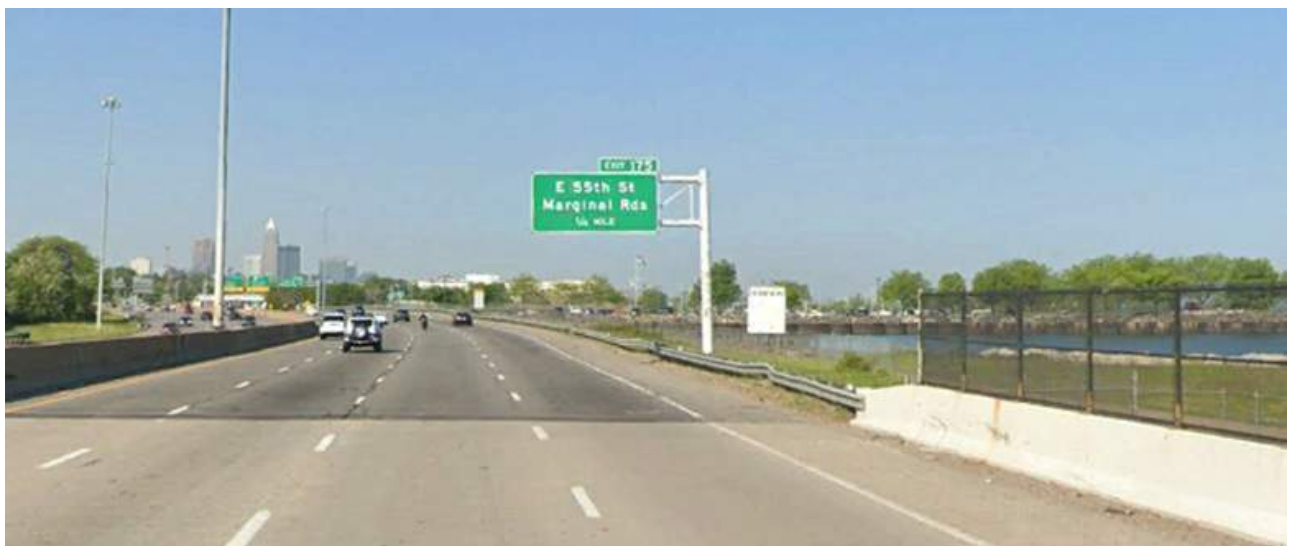
Figure 60: QWS-OVRHD-D12-I-90_WB AT DOWNTOWN Street view of Proposed QWS Lite on existing cantilever sign
