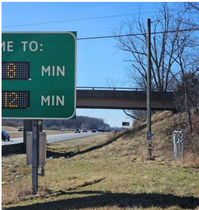
Figure 12: QWS-D5-I-70_WB Existing DDMS with existing detection camera attached to back of sign
