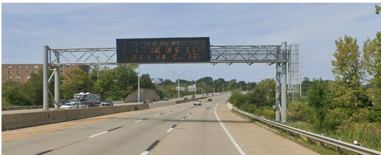
Figure 72: QWS-GRND-D12-OH-176_NB AT STEELYARD Street view of existing DMS sign and structure to be replaced with new
