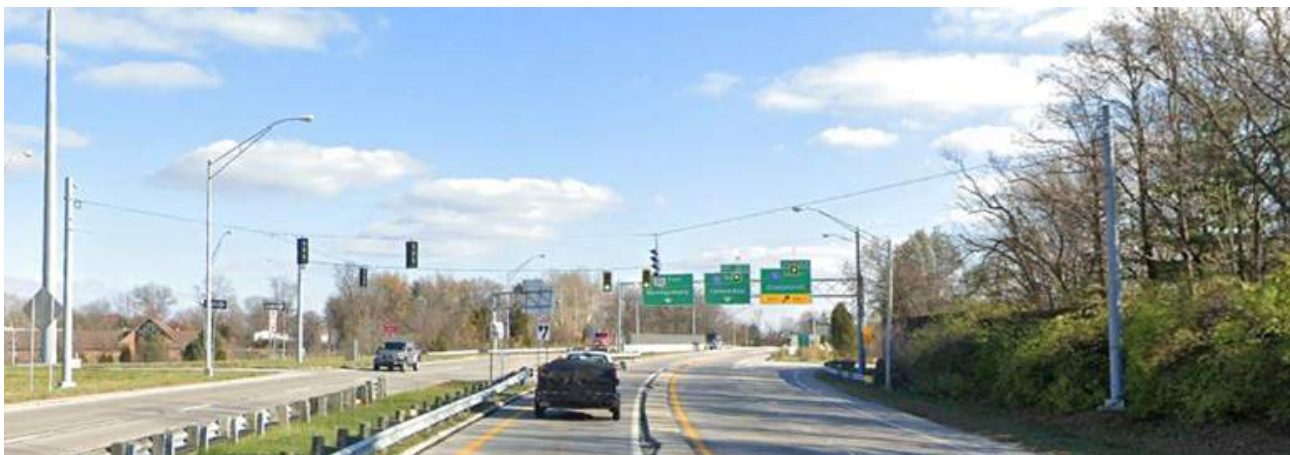
Figure 48: QWS-OVRHD-D8-OH-126_EB AT I-71 street view detection camera proposed location on existing traffic signal at the I-71 off-ramp
