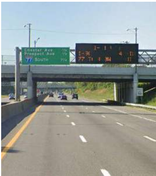
Figure 66: QWS-OVRHD-D12-I-90_WB AT DOWNTOWN Street View existing cantilever structure to be replaced with static sign truss structure and location of proposed detection camera pole.
