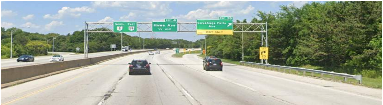
Figure 8: Street View: LITE-D4-OH-8_NB AT HOWE AVE Street view of proposed QWS Lite sign on existing truss structure adjacent to the North SR 8/East SR 59 guide sign
