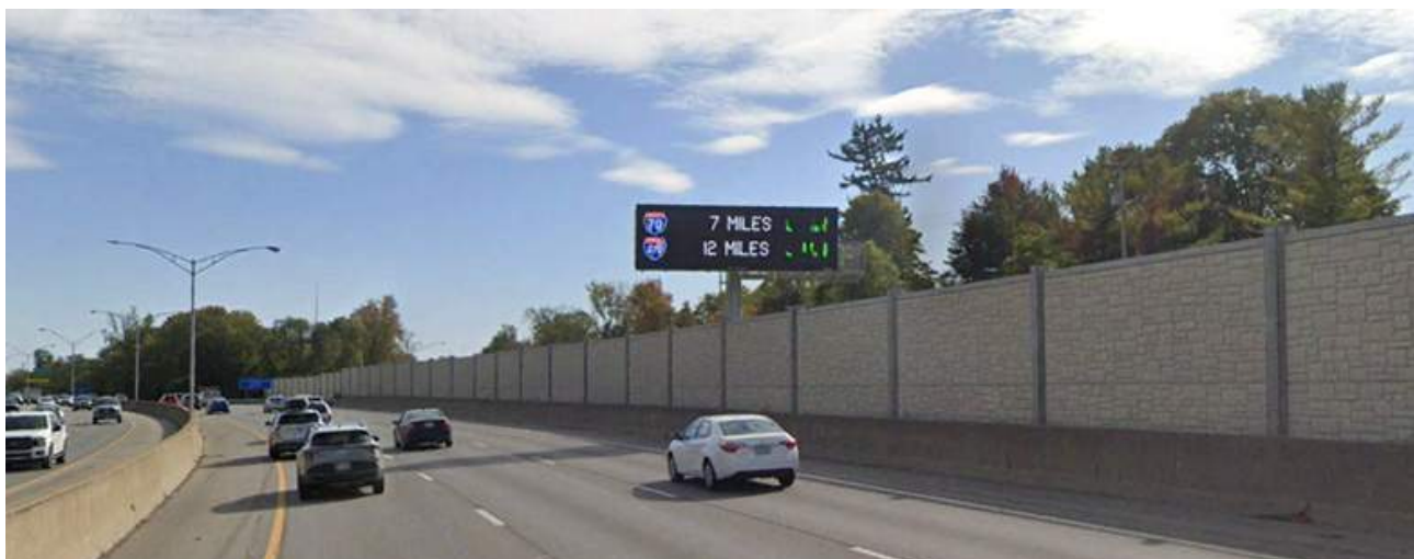
Figure 33: QWS-GRND-D6-OH-315_SB AT IR-670 street view of existing DMS Location
