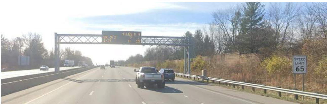
Figure 44: QWS-OVRHD-D8-I-71_SR 126 street view of existing DMS (to be replaced)
