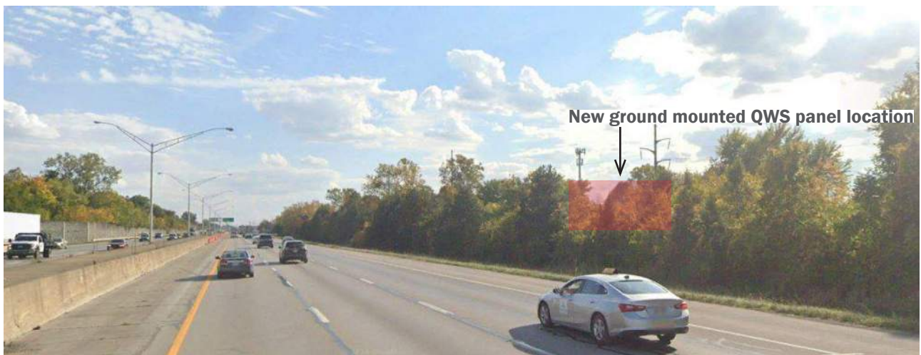
Figure 19: QWS-GRND-D6-I-71_SB AT MORSE RD view of proposed ground mounted QWS panel located at SLM 24.12 SB at Morse Rd on the right-hand side of the road
