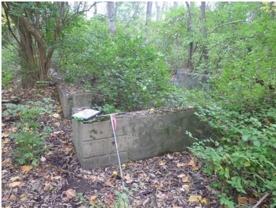
Photo Location 11: Abandoned structure foundation, facing southeast.
