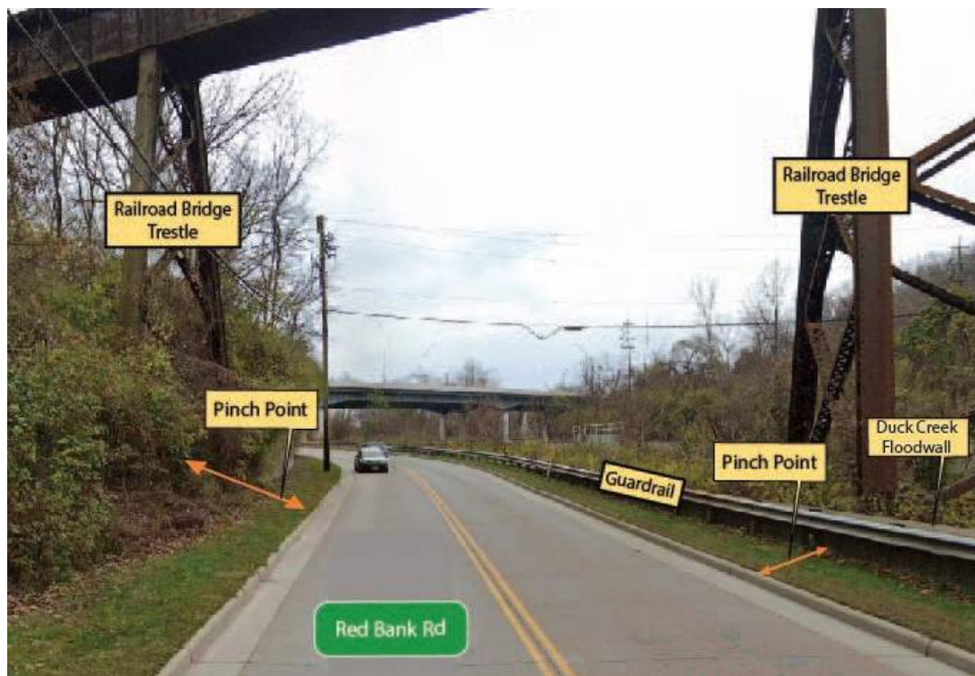
Figure 3: Pinch point between Railroad Bridge Trestles, the Duck Creek Floodwall, and Red Bank Road, facing south (Google Maps, 2022).
