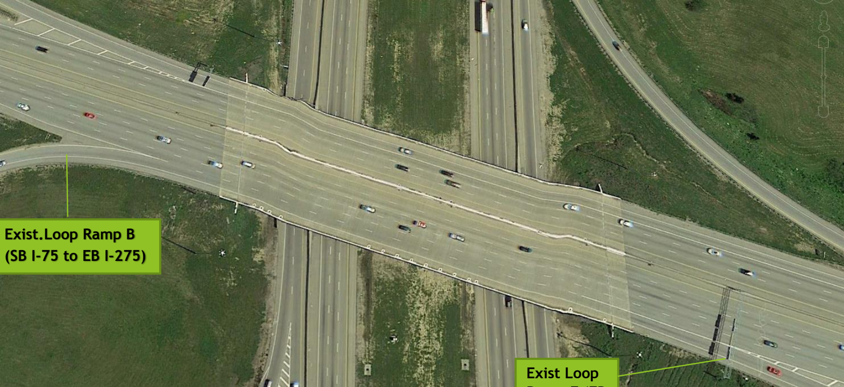
Close-up of EB I-275 weaving area.
