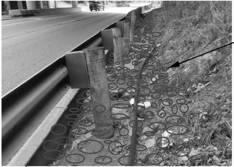
PLACE GEOTEXTILE FABRIC AND TYPE 'D' ROCK BEHIND CURB, AND AROUND/BEHIND GUARDRAIL POSTS TO PREVENT FURTHER EROSION THE FOLLOWING QUANTITIES HAVE BEEN CARRIED TO THE GENERAL SUMMARY:
