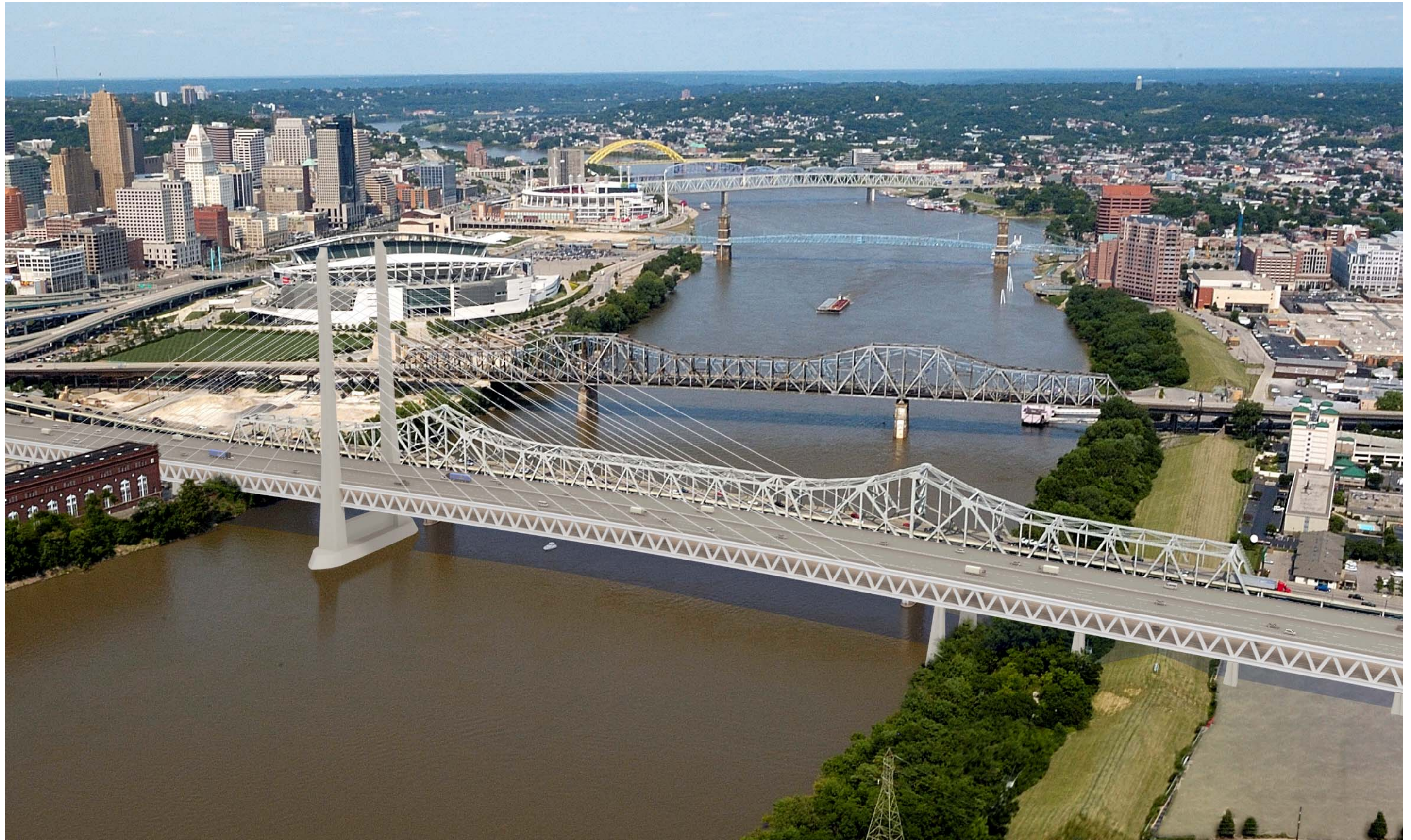
ALTERNATIVE 6 – ONE TOWER CABLE STAYED
