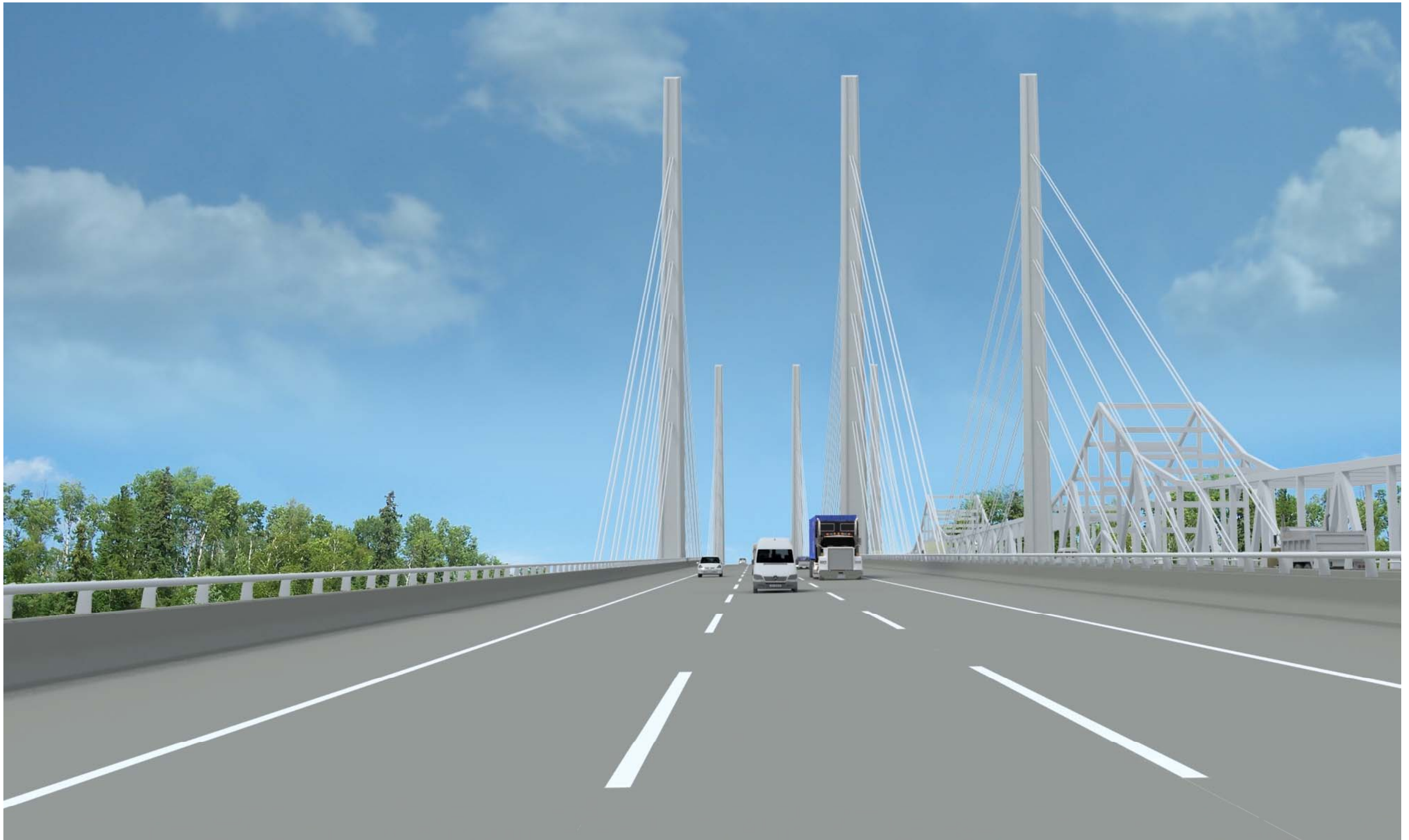
ALTERNATIVE 3 – TWO TOWER CABLE STAYED
