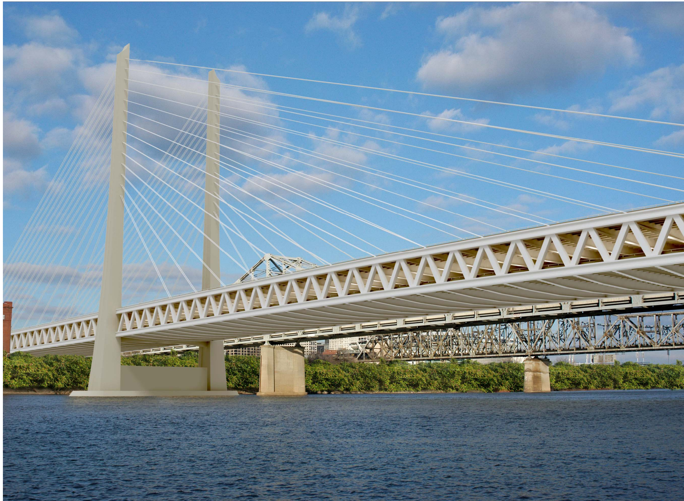
ALTERNATIVE 6 – ONE TOWER CABLE STAYED
