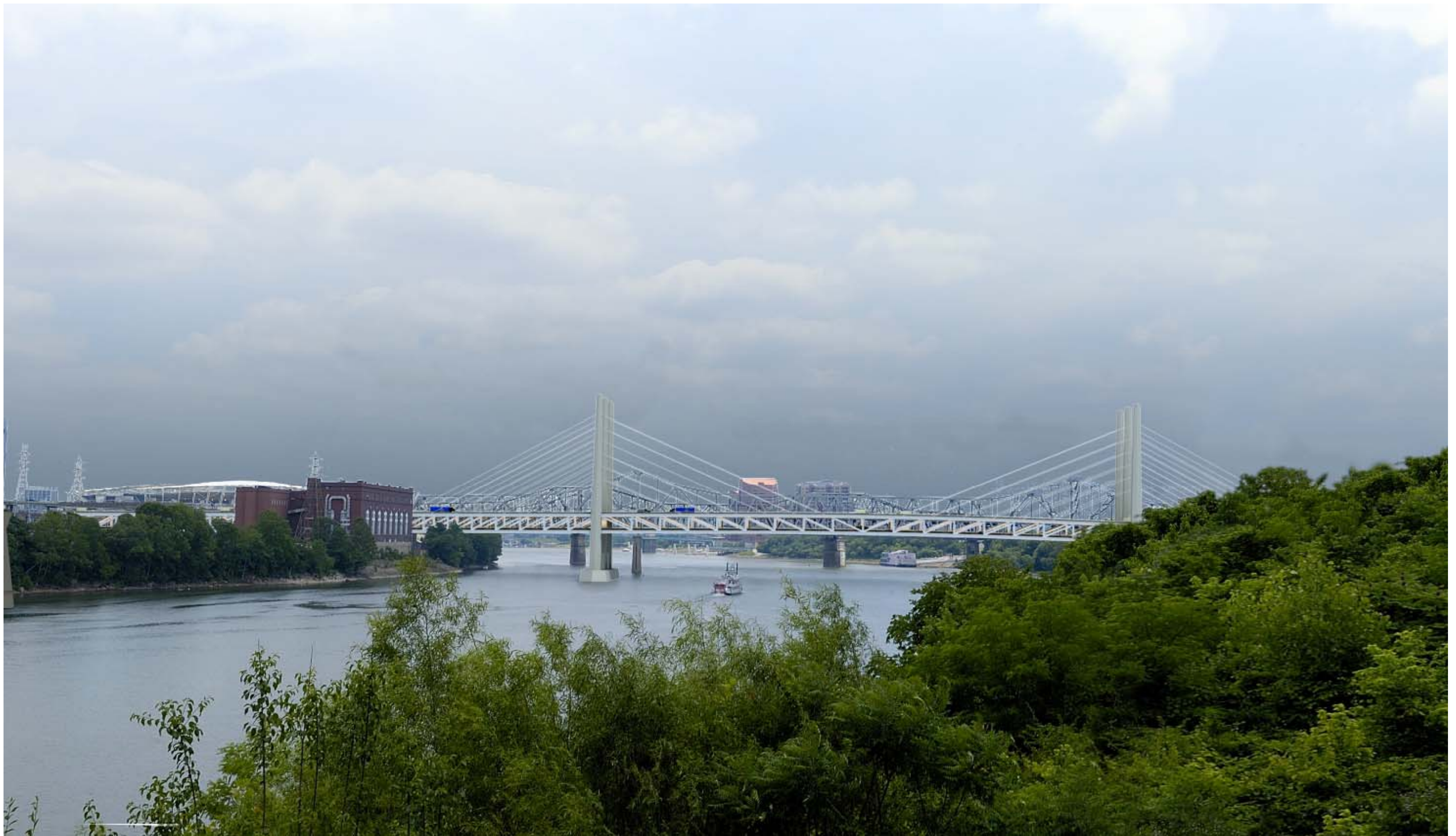
ALTERNATIVE 3 – TWO TOWER CABLE STAYED
