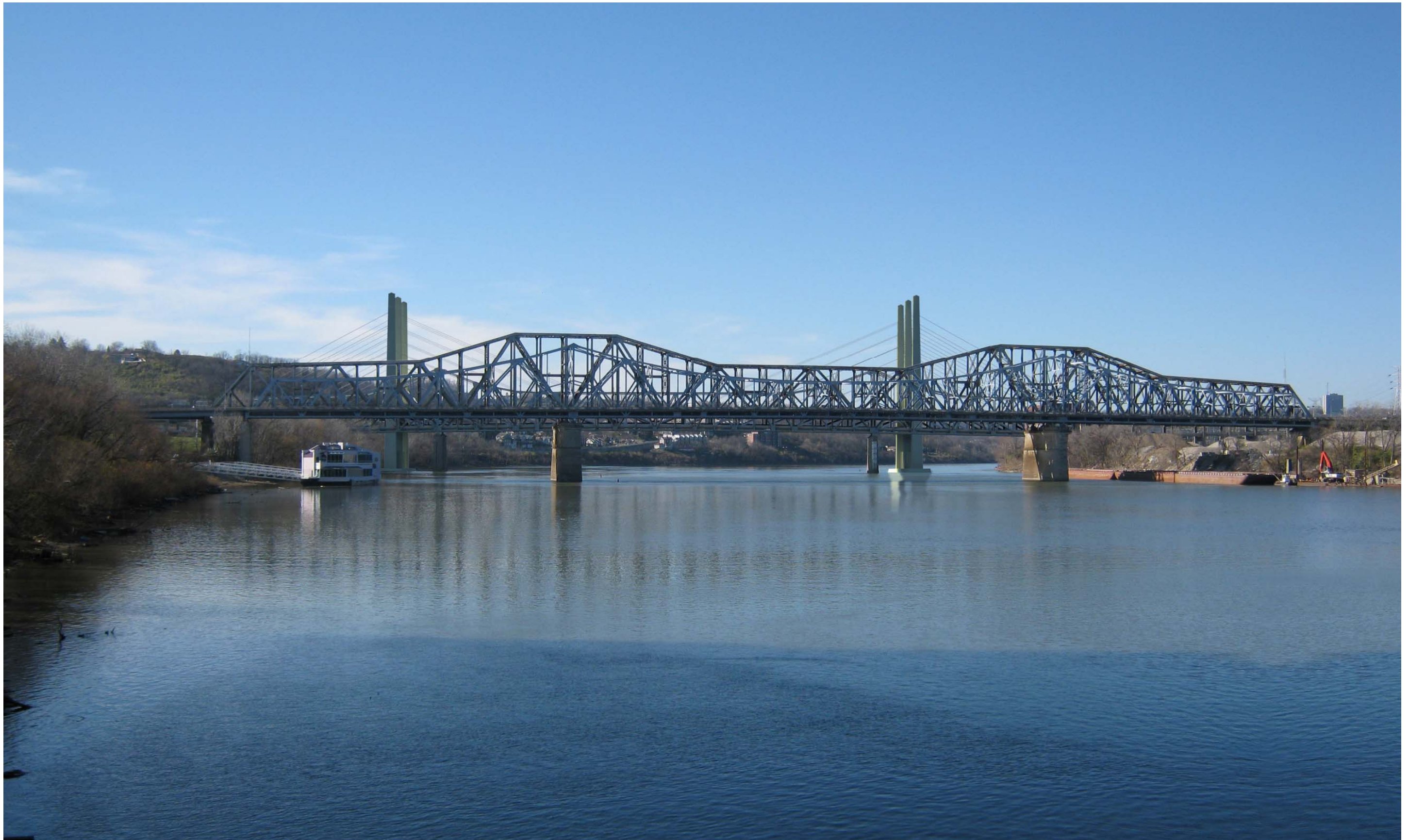
ALTERNATIVE 3 – TWO TOWER CABLE STAYED
