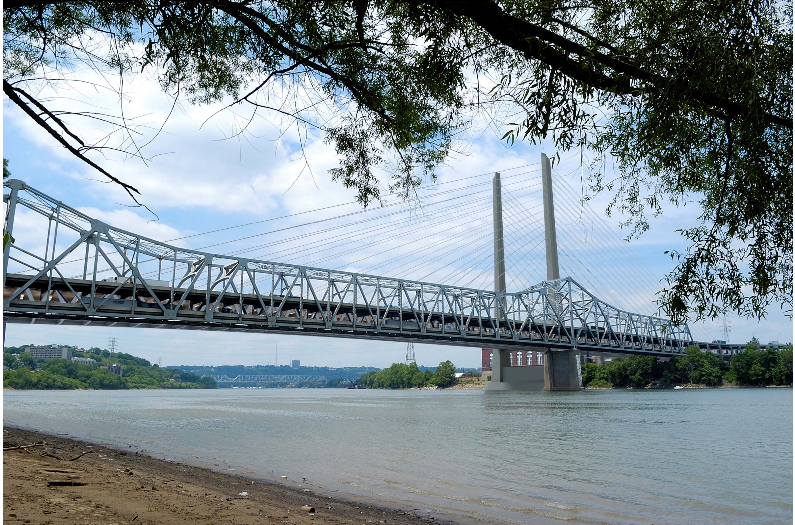
ALTERNATIVE 6 – ONE TOWER CABLE STAYED
