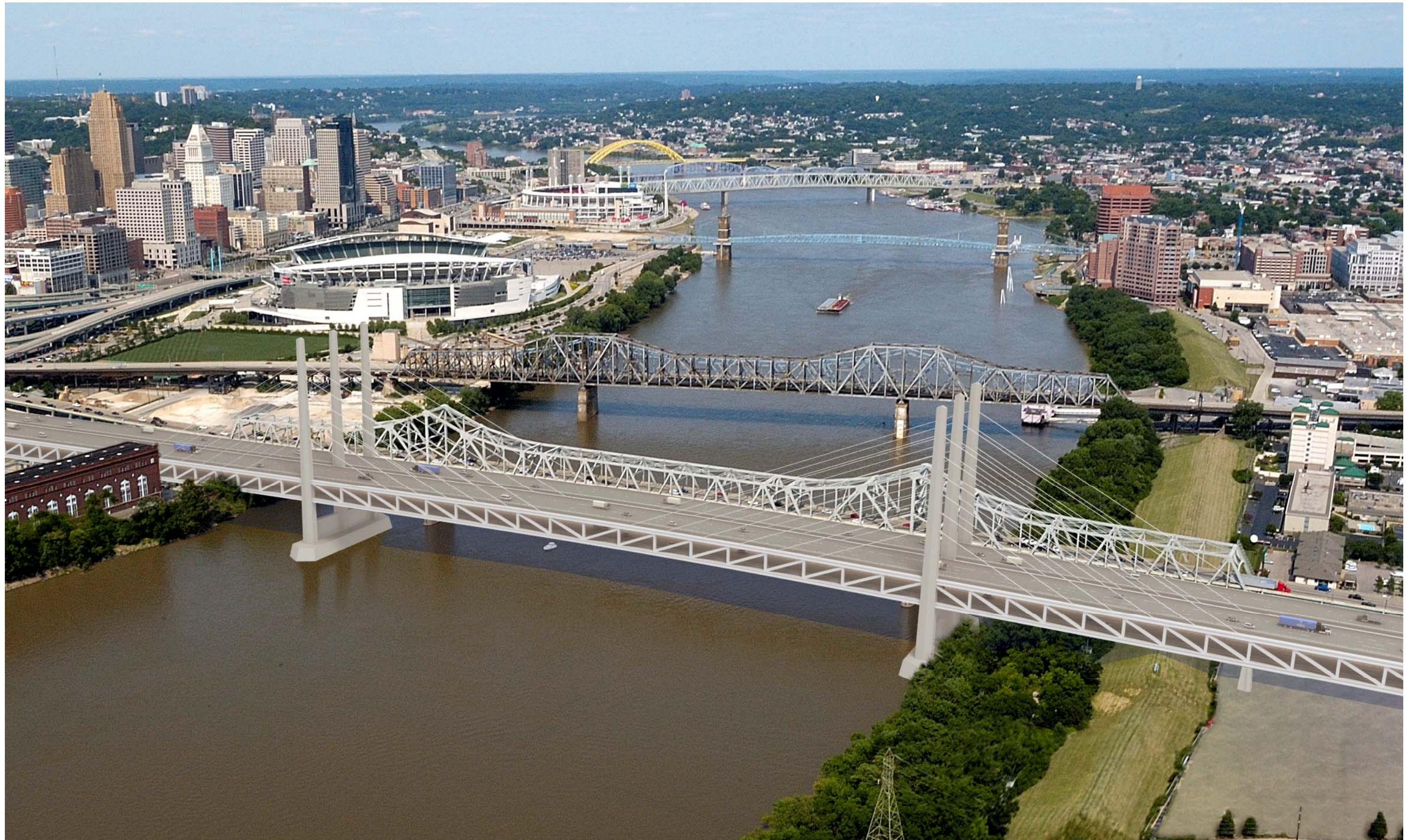
ALTERNATIVE 3 – TWO TOWER CABLE STAYED
