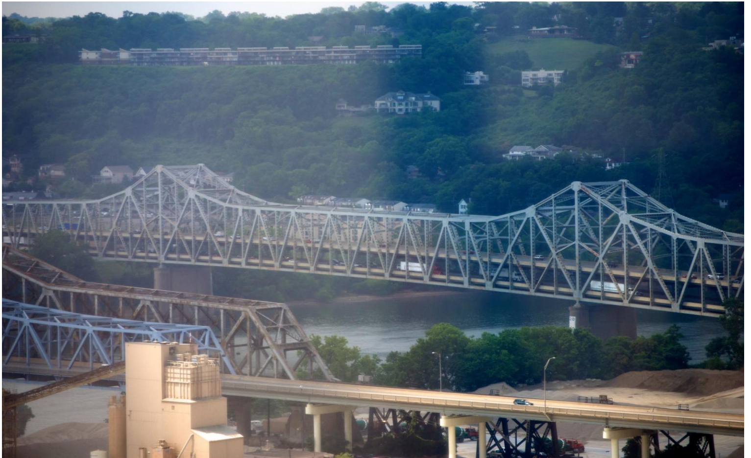
Photographs of the Brent Spence Bridge Site
