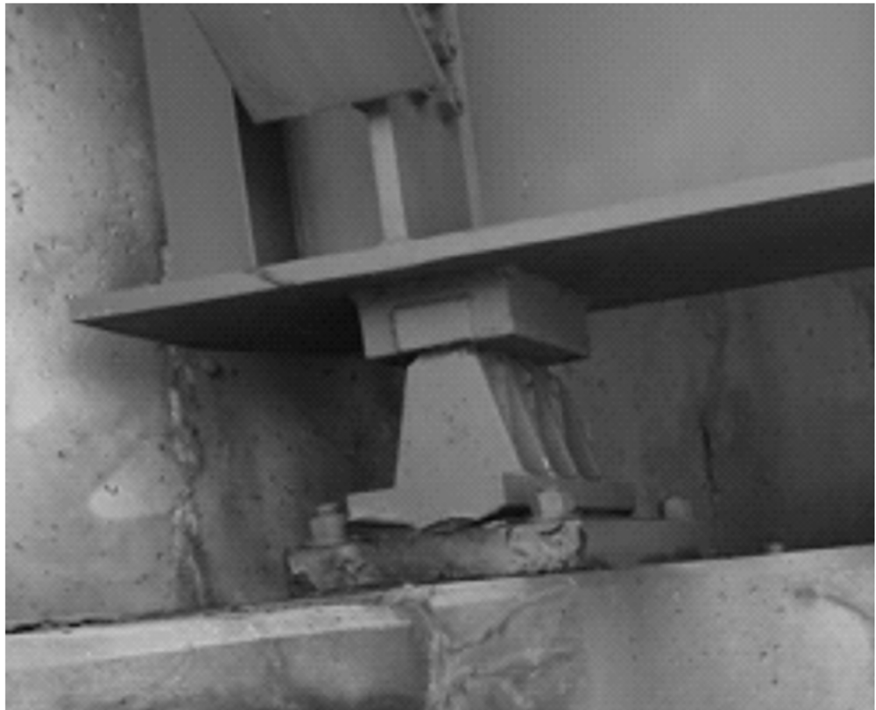
TYPICAL ABUTMENT BEARING
