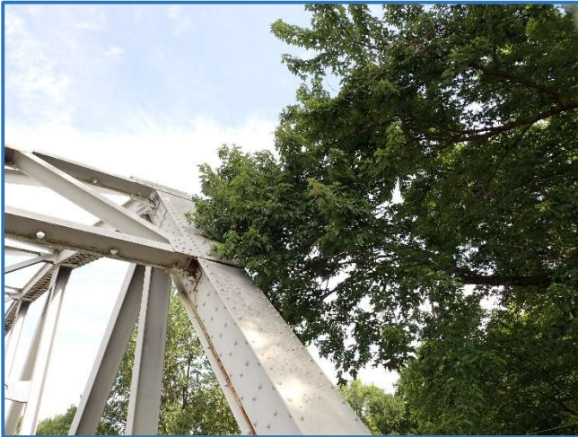
Photo 95 - Tree encroaching on end post in Span 3, North Truss, between Panel Points 9 and 10, looking northwest
