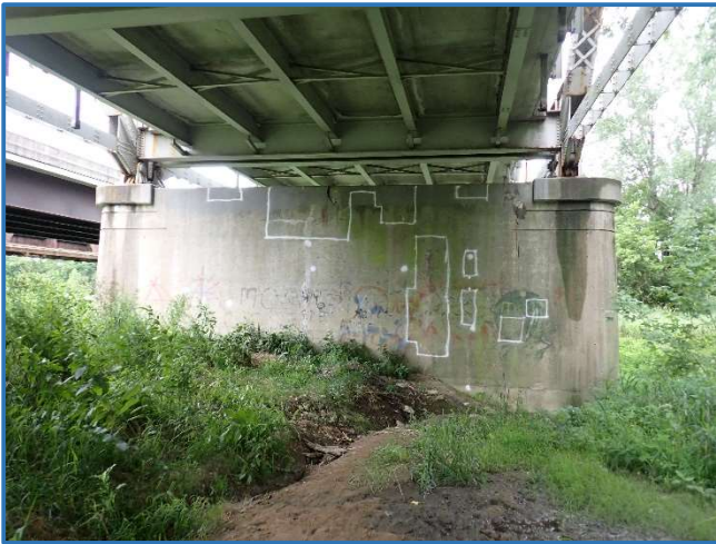
Photo 82 - East face of Pier 4
