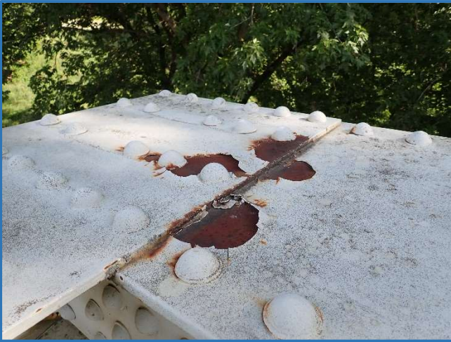
Photo 25 - Typical paint spot failure on top of upper chord, with active corrosion. Shown Span 4, North Truss, east of U1, looking northwest
