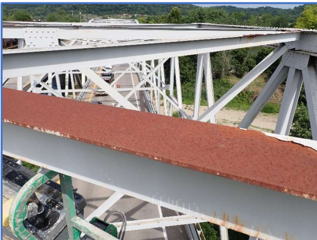
Photo 63 - Upper lateral bracing paint failure with surface corrosion. Shown is worst case in Span 3, North Truss, between Panel Points 5 and 6, looking southeast
