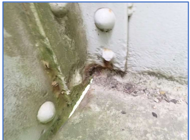
Photo 53 - Up to 50% section loss in rivet heads in Span 3, Floorbeam 4, gusset plate clip angle connection, south end, looking west
