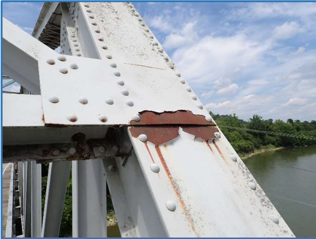
Photo 35 - Paint failure with surface corrosion on top face of end post in Span 1, North Truss, between Panel Points 7 and 8, looking west
