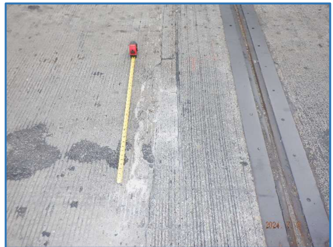
Photo 91 - Spalling in west approach slab, just west of rear abutment, looking north
