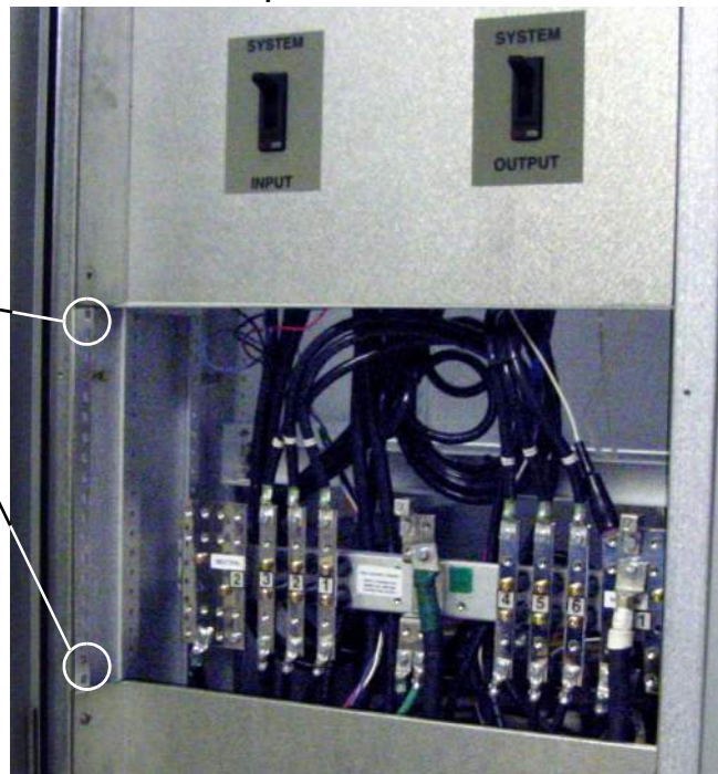
Figure 15 Maintenance Bypass Cabinet—access plate removed
