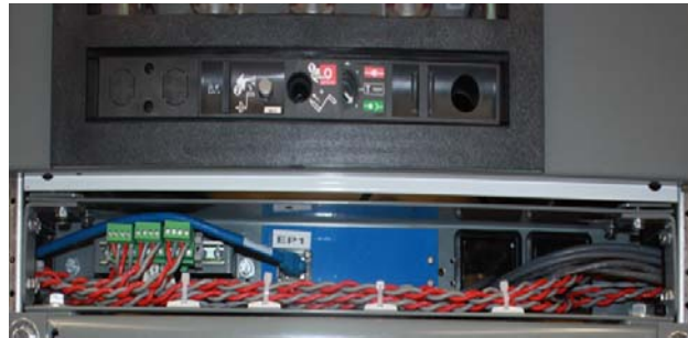
Figure 40: Example of Ethernet Modbus TCP Cable (Blue) Connection to Labeled Ethernet Port
