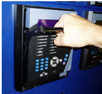
FIGURE 3-8: Rotate Handle to Stop Position
