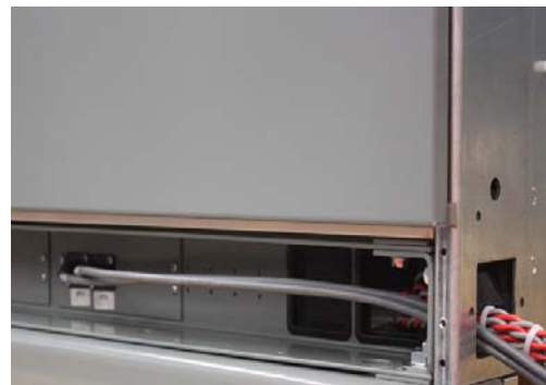
Figure 37: ULP Cables routed and connected to labeled ULP ports in adjacent section wireway
