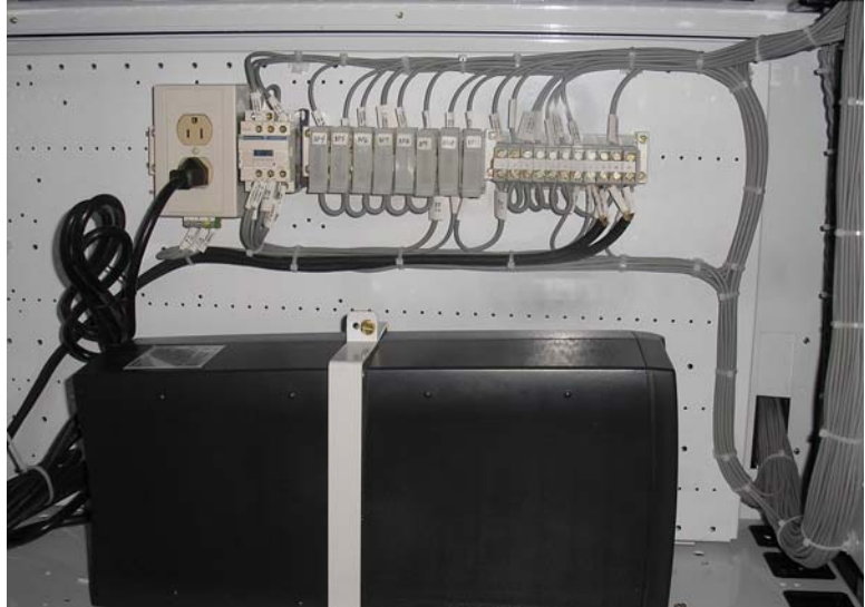
Figure 14: UPS Assembly
