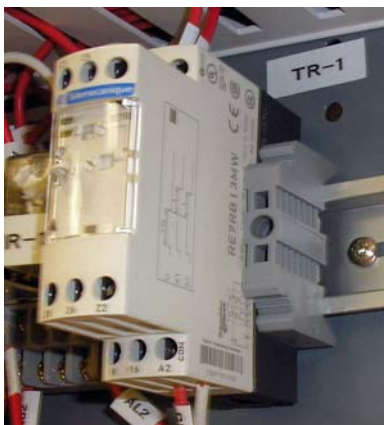
Figure 20: Generator Start Relay
