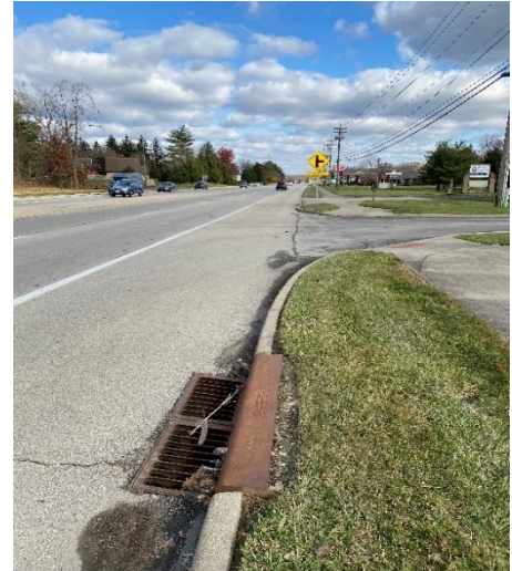
Photo 2 – Inlet at curb line
