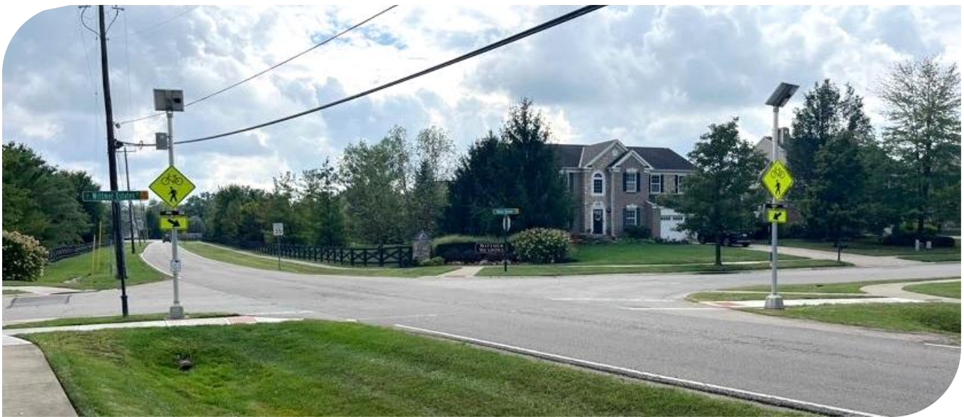
Figure 57. An RRFB is present at the intersection of Mt Zion Road, Wittmer Meadows Drive, and Wittmer Estates Drive
