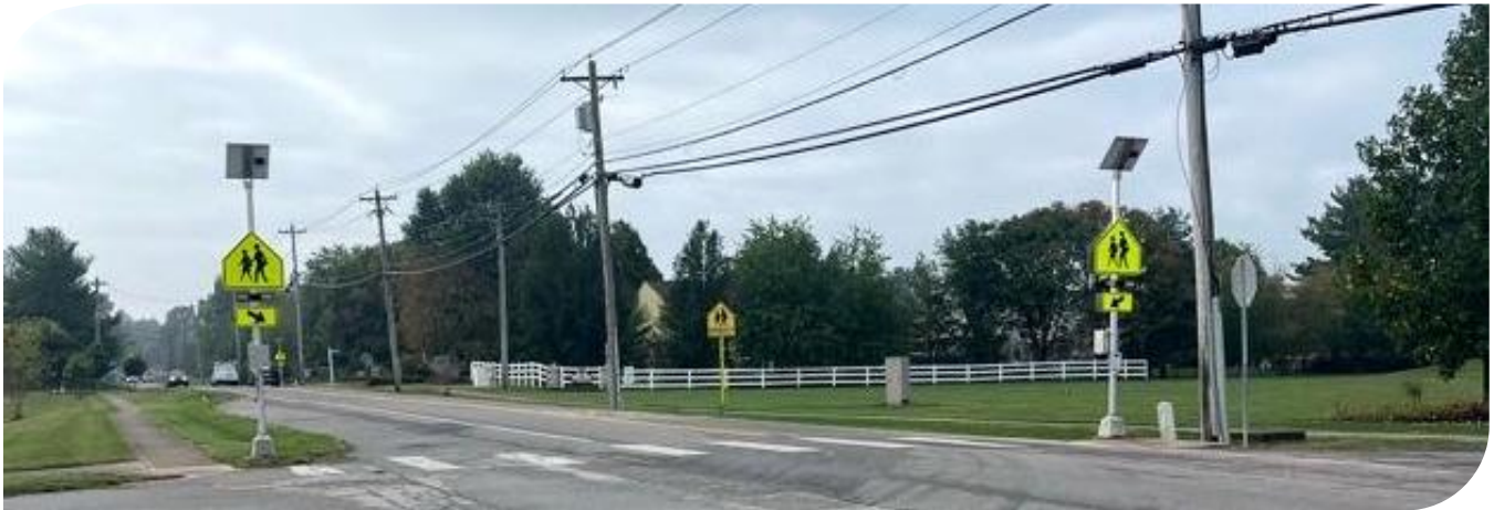
Figure 63. RRFB and high-visibility cross on Buckwheat Road at the school's south entrance
